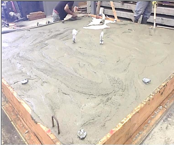
Figure (3.11): Sandwich Slab Specimen after Placing the High-Strength Mortar
