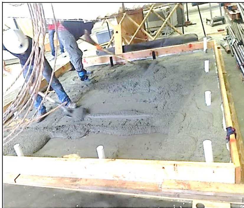
Figure (3.10): Pouring of High-Strength Mortar at UCI SETH Laboratory
