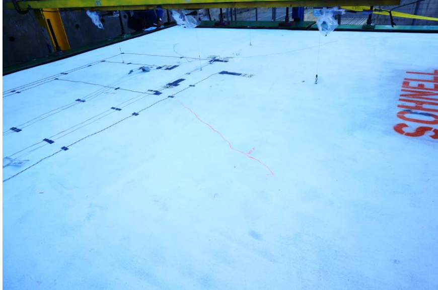
Figure (3.54): First Hair Crack on the Tension Top Side of Sandwich Slab Specimen C at a Load Level of about 6.0 kips (26.7kN)
