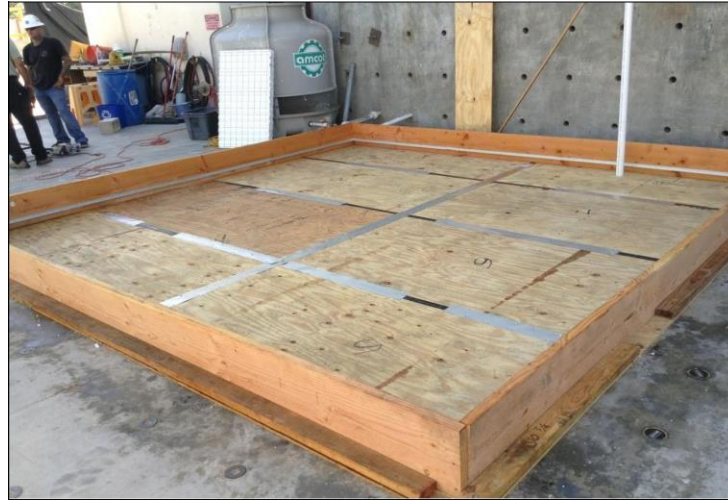
Figure (3.22): Plywood Frame on which Slabs were Casted
