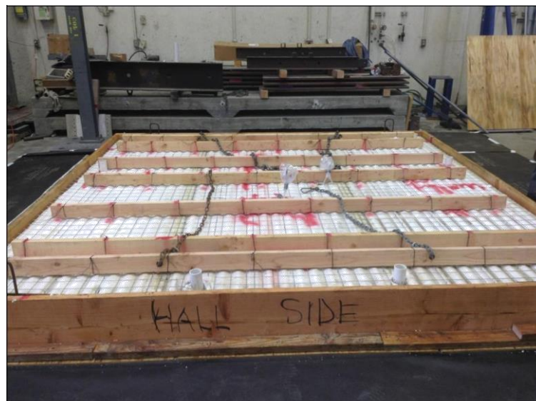
Figure (3.23): Plywood Casting Frame after Polystyrene with Steel Mesh was Placed
