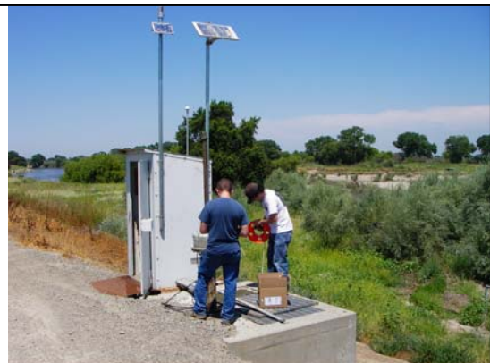
DO-31 New Jerusalem Drain Student intern and Justin Graham using bucket to sample down manhole over New Jerusalem Drain.
