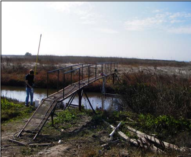
DO-20 Los Banos Creek Student Intern Sampling near recently completed bridge.
