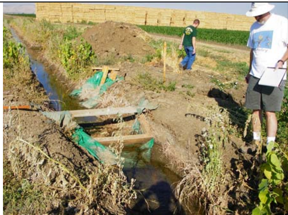
DO-101 WFP-UD-IN Will Stringfellow looking at weir structure at start of un-vegetated ditch on Westside Patterson Farms.
