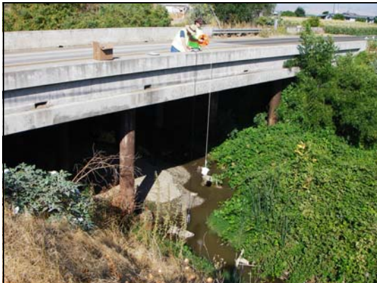
DO-54 Los Banos Creek at Ingomar Student intern taking samples from bridge over Los Banos creek.
