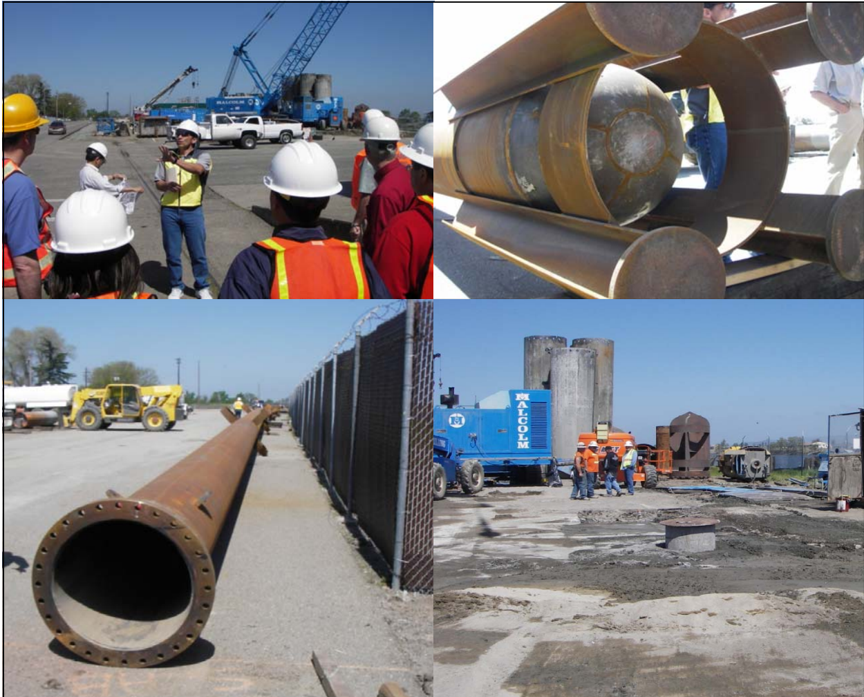
Port of Stockton Photos of tour of Dissolved Oxygen Aeration Facility.
