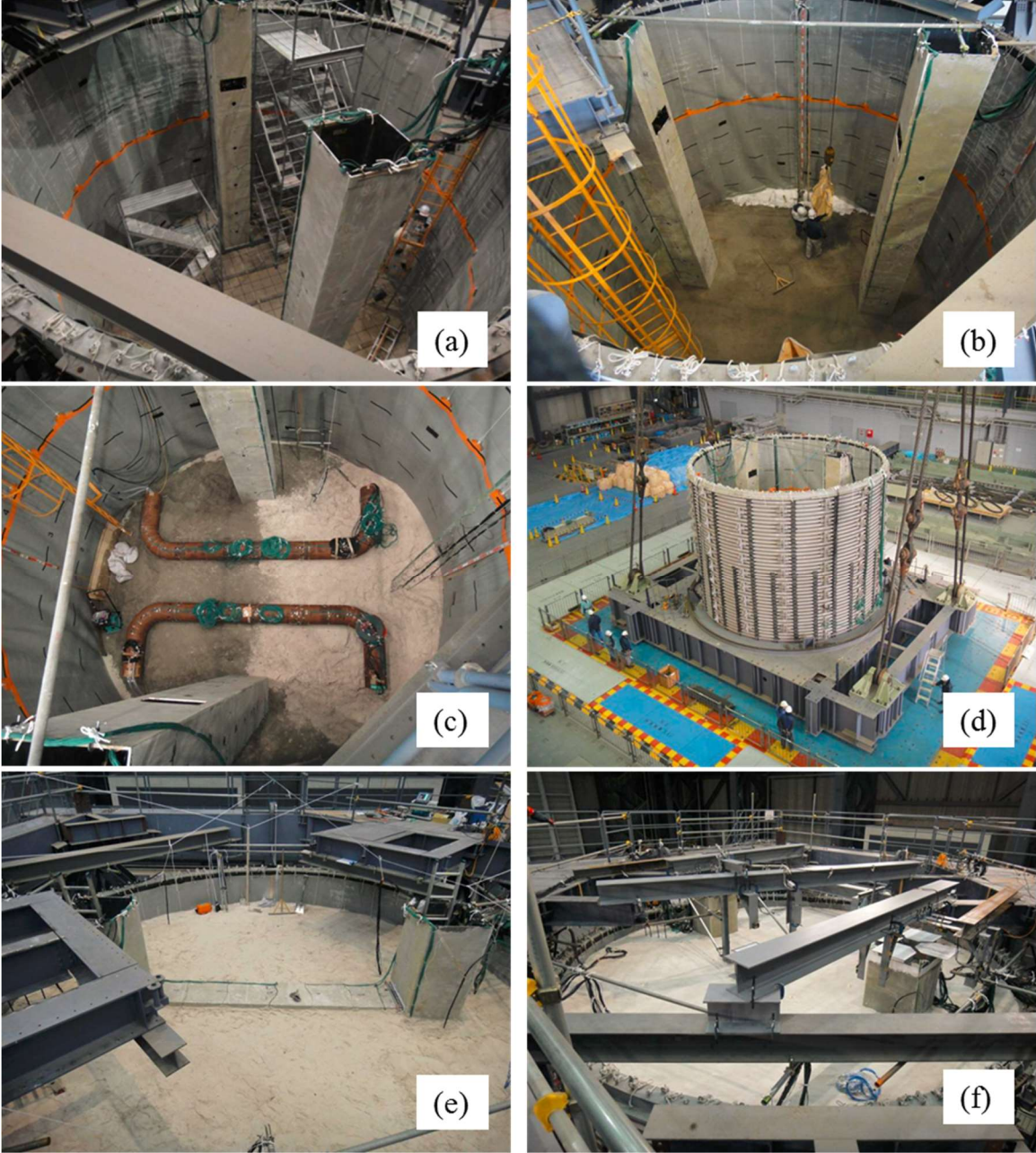
Figure 2.3. Assembly stages of the test specimen
