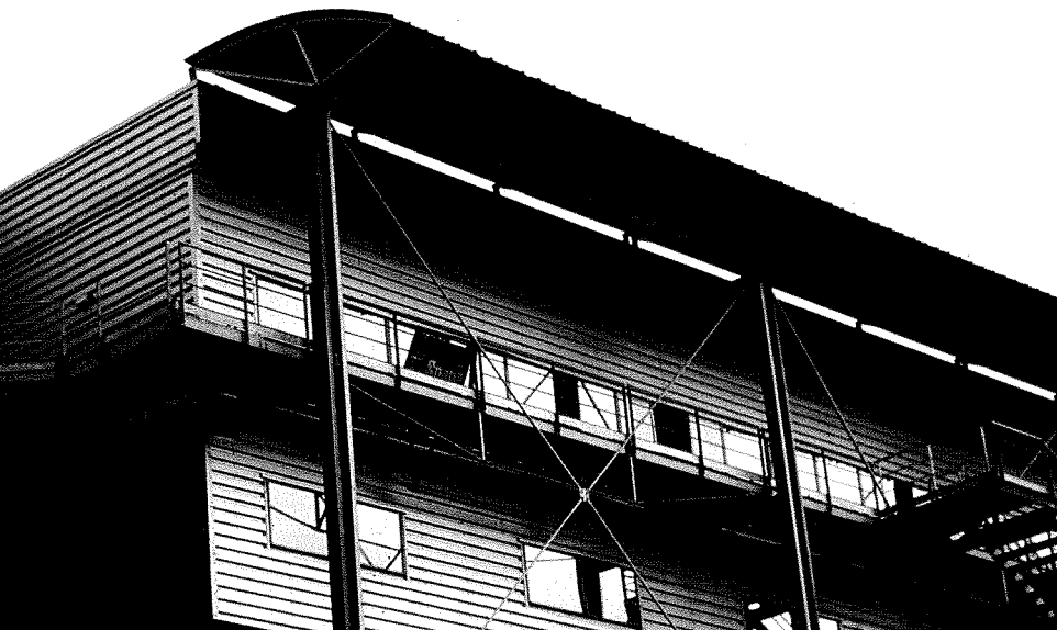
Hôtel industriel Pantin, a similar project outside Paris. Design by Paul Chemetov and Borja Huidobro.
