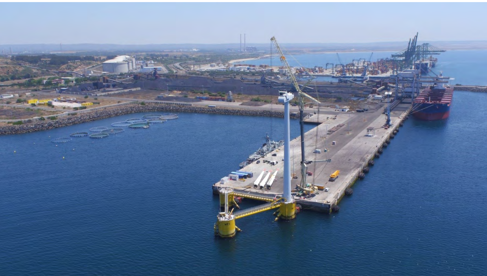
Decommissioning of Principle Power's 2 MW prototype floating turbine after five years of operation in the Atlantic Ocean. Porto de Sines, Portugal, July 2016. Photo: Principle Power
