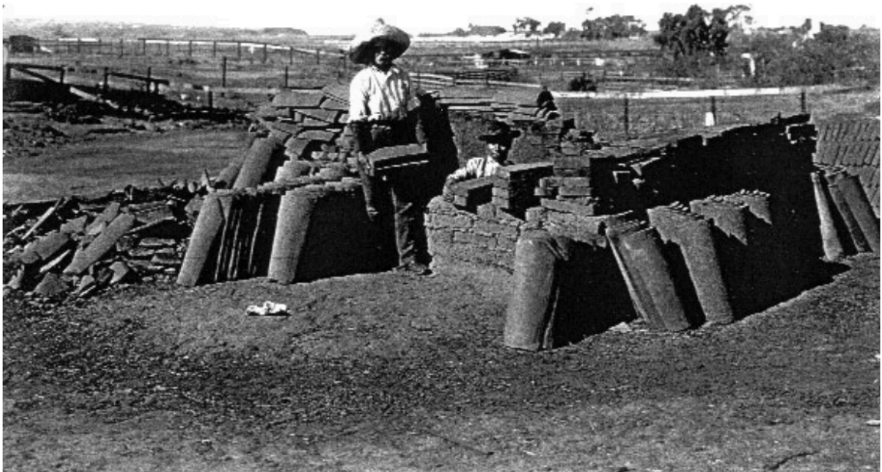
Figure 4.11: Workmen dry adobe bricks during the site’s renovation ~1908-1909. From V. A. Walsh, 2004, Una casa del pueblo—A town house of old San Diego , The Journal of San Diego History , 50(1/2), p. 9. Copyright by San Diego Historical Society, #2387. Reproduced under Fair Use in accordance with the Visual Resources Association’s Statement on the Fair Use of Images for Teaching, Research, and Study (2013, pp. 11-12).
