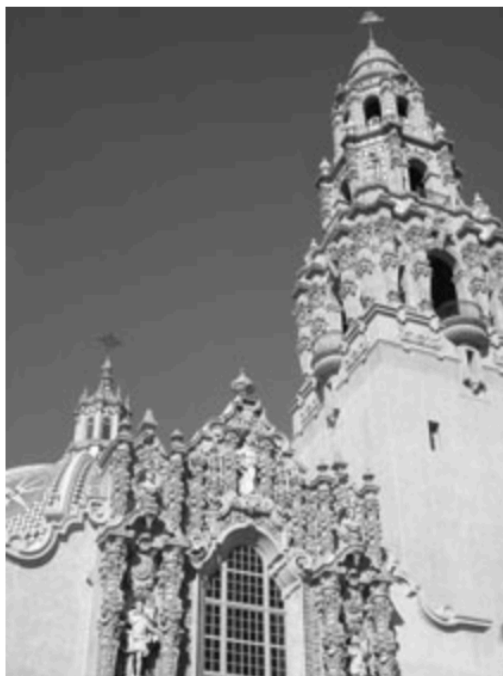
Figure 4.17: 1915 image of Goodhue's ornate California Quadrangle building, an architectural highlight of the park. From J. Bechtol, 2009, 1915 Panama-California Exposition, retrieved from https://public.csusm.edu/becht004/1915expopage.html Previously published on January 1, 1915 in the San Diego Union . Reproduced under Fair Use in accordance with the Visual Resources Association's Statement on the Fair Use of Images for Teaching, Research, and Study (2013, pp. 11-12).
