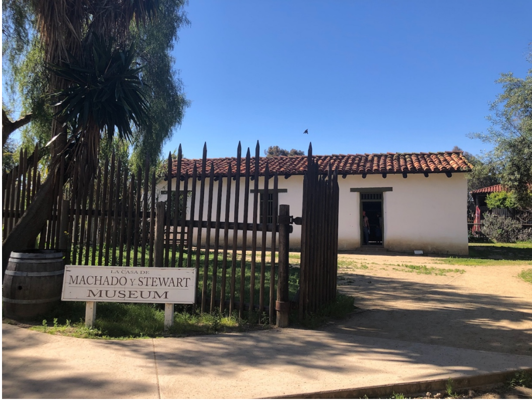
Figure 7.7: Exterior of La Casa de Machado y Stewart Museum within Old Town San Diego State Historic Park. Photo by author, 2019.
