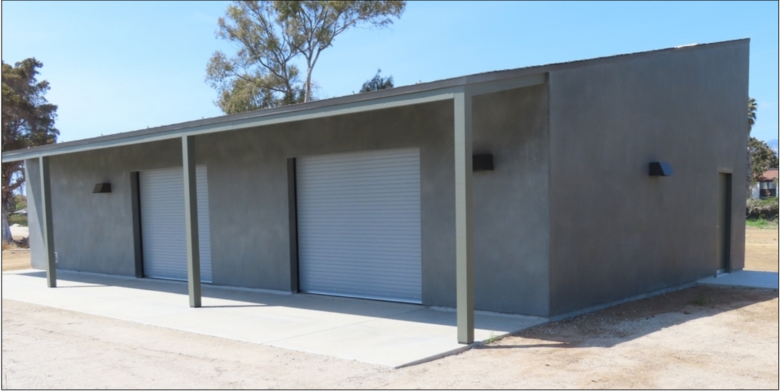
The completed "Gator Barn", or ROOST (Restoration, Outreach and Open Space Toolshed) at NCOS.
