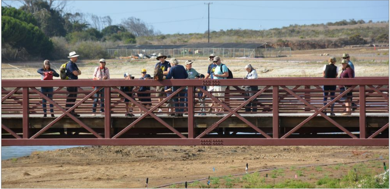
NCOS visitors on the long bridge across the eastern arm of the wetland.
