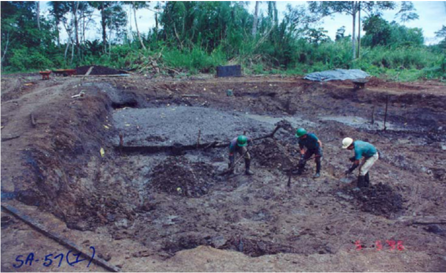
FIGURE 29 Oil well Sacha-57 (pit #1) during Texaco's remedial action plan (RAP). Taken by Woodward-Clyde (the environmental remediation contractor) on May 5, 1996, the photo depicts heavy crude embedded at the bottom of the pit after liquids and viscous hydrocarbon contents were removed. Source: Maria Aguirre Salazar y Otros v. ChevronTexaco Corp. , Case No. 002-2003-P-CSJNL (2011-63-1), p. 11,849, Provincial Court of Justice of Sucumbíos, Nueva Loja, Ecuador.
