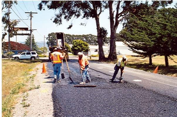
Figure 5.3: Overlay placement (MB4-G).
