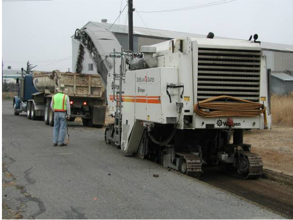
Figure 2.5: Milling of existing roadway
