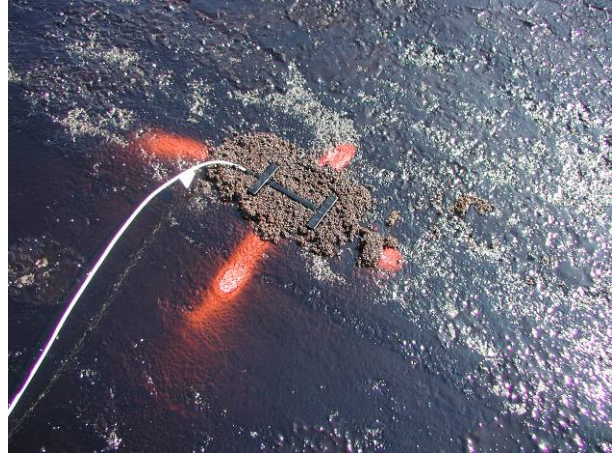
Figure 2.12: Installation of strain gauges
