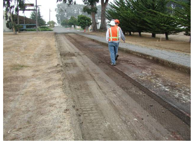
Figure 2.6: Exposed subgrade
