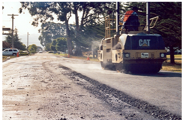
Figure 5.2: Overlay compaction (AR4000-D).
