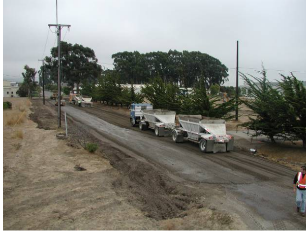
Figure 2.10: Base construction
