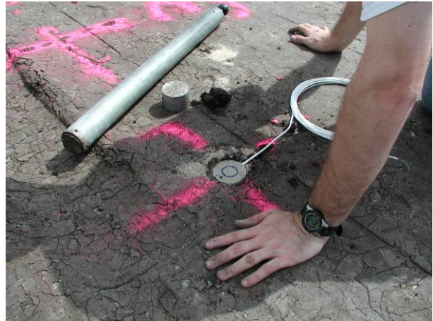
Figure 2.9: Installation of pressure cell
