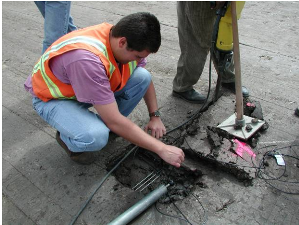
Figure 2.8: Installation of Time Domain Reflectometer
