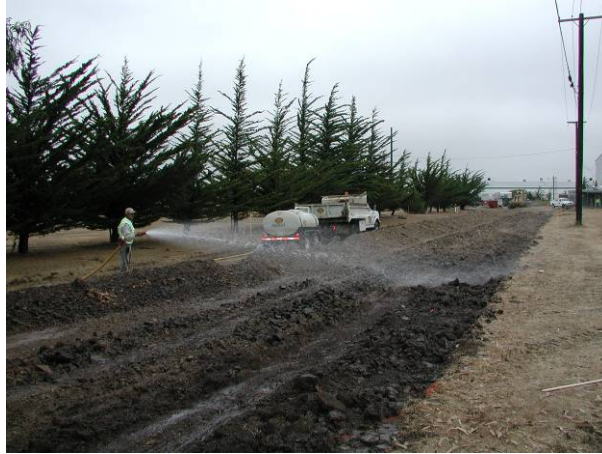
Figure 2.7: Subgrade preparation
