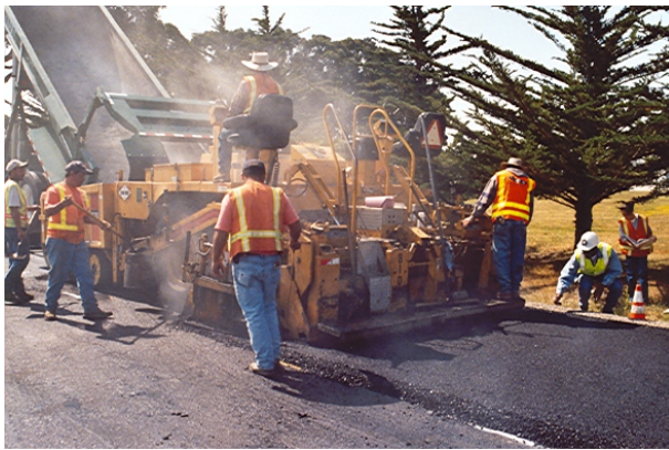
Figure 5.1: Overlay placement (RAC-G).
