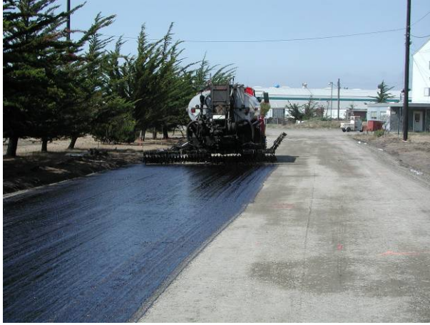
Figure 2.11: Base priming
