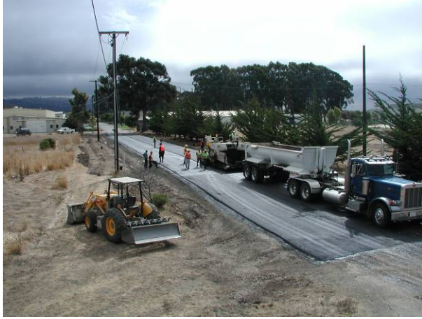
Figure 2.13: Asphalt concrete placement
