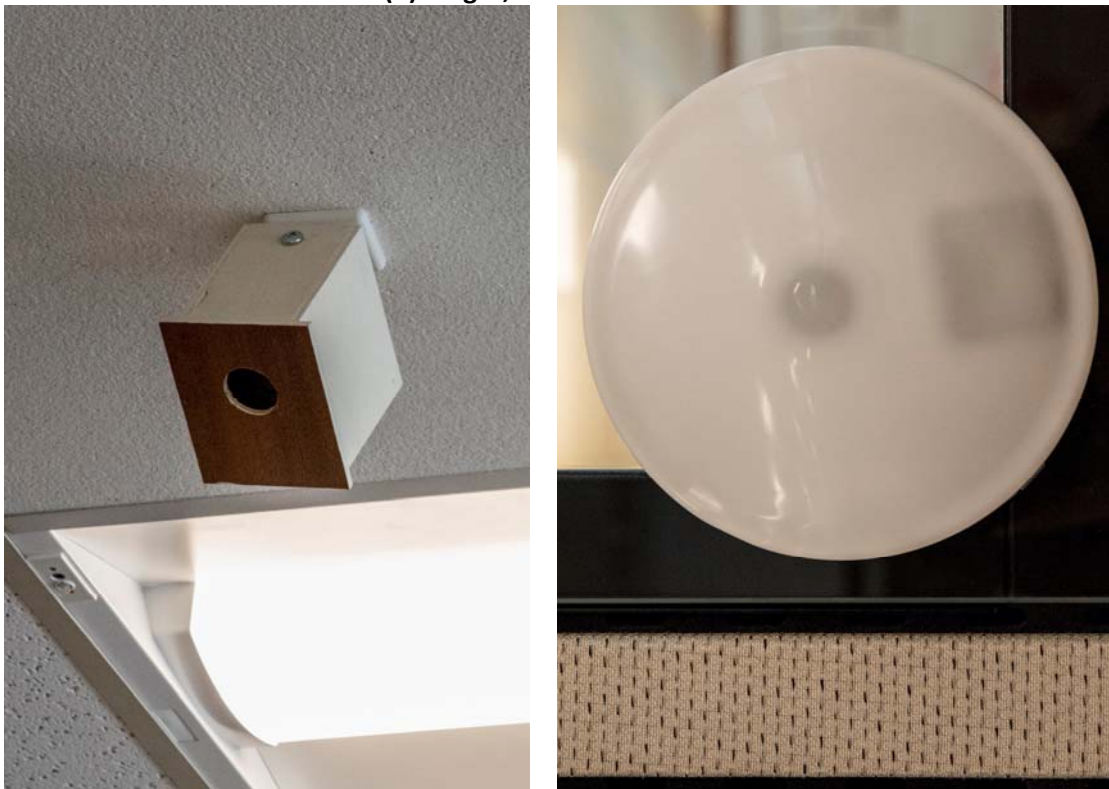
Figure 6: Cubicle Occupancy Sensors, Technology Package 2(a) – left, installed in ceiling – and 2(b) – right, furniture mounted
