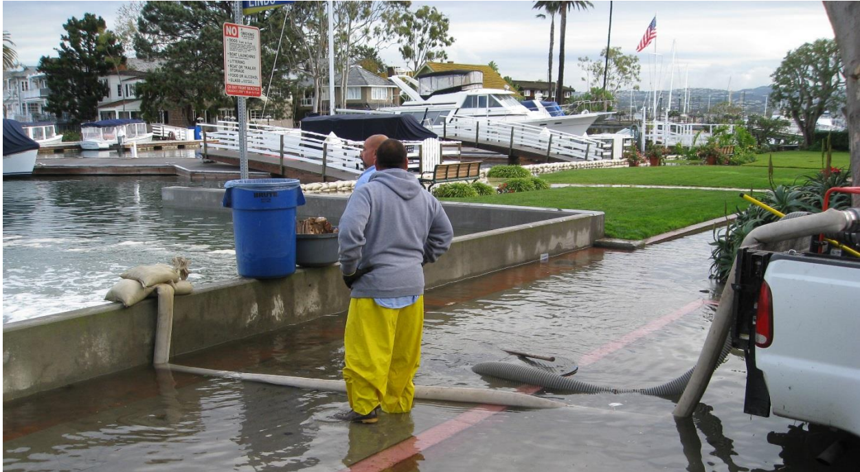
Figure 1.2. Wave overtopping seawall in the lower peninsula of Newport Beach in December 2012.
