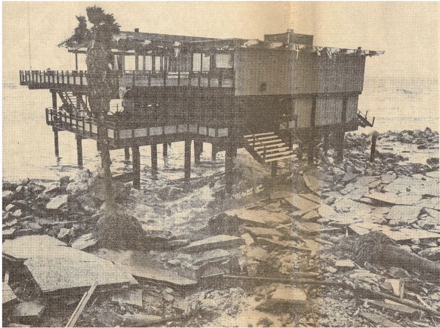
Figure 2.7 Beach erosion extended beneath the Santa Barbara Yacht Club in March 1983 (source: Santa Barbara News-Press).
