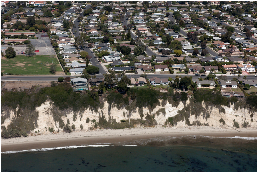
Figure 2.16 A number of homes along the Mesa are within 15 meters (49 feet) of the cliff edge (photo: Kenneth and Gabrielle Adelman, California Coastal Records Project).
