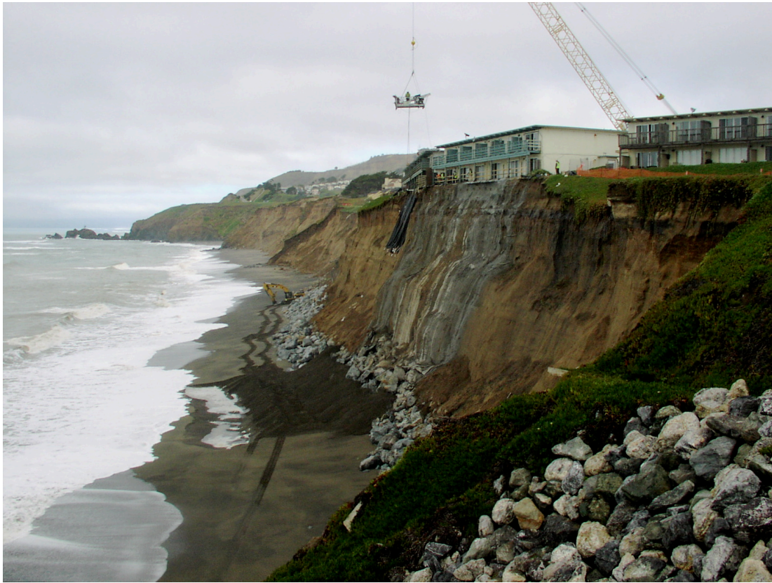
Figure 1.3 Apartments in Pacifica, California were threatened by wave attack during the winters of 2009-2010 and 2010-2011 and subsequently evacuated.
