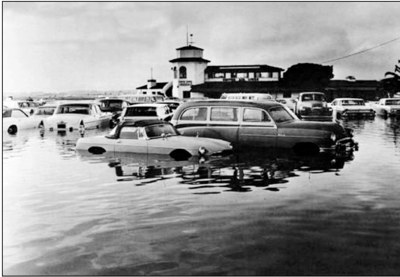
Figure 2.2 The Santa Barbara Airport parking lot flooded in 1969 (source: Santa Barbara Airport).
