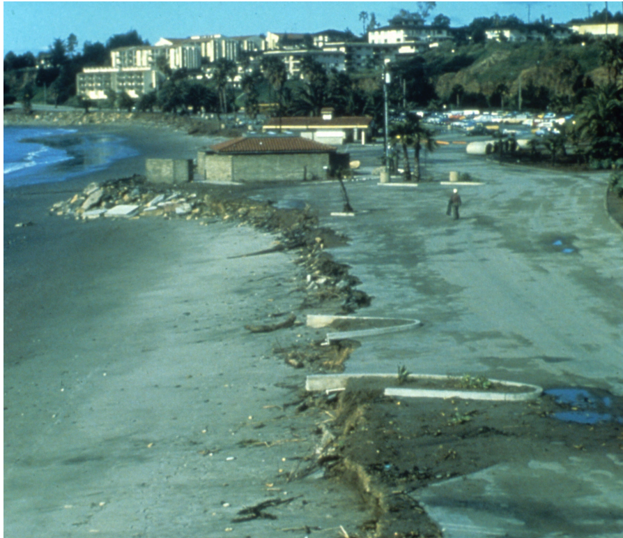
Figure 2.8 Erosion removed part of the Leadbetter Beach parking lot during the 1983 El Niño.
