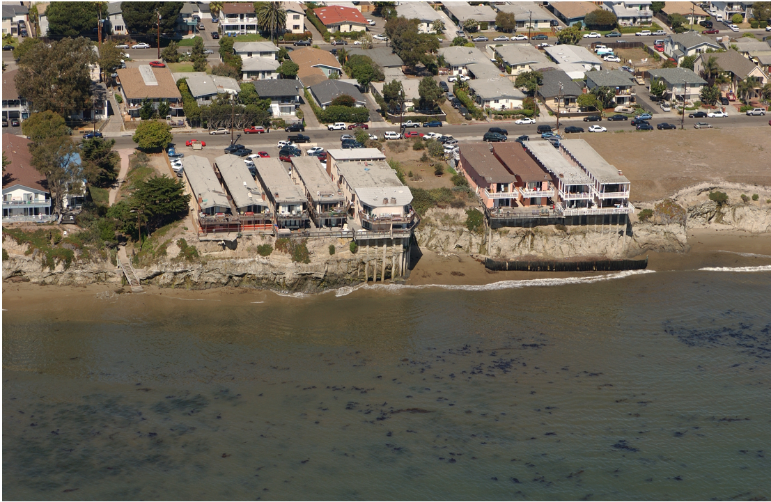
Figure 1.2 Undercut apartment buildings in the Isla Vista area of Santa Barbara County, California (photo: Kenneth and Gabrielle Adelman, California Coastal Records Project).
