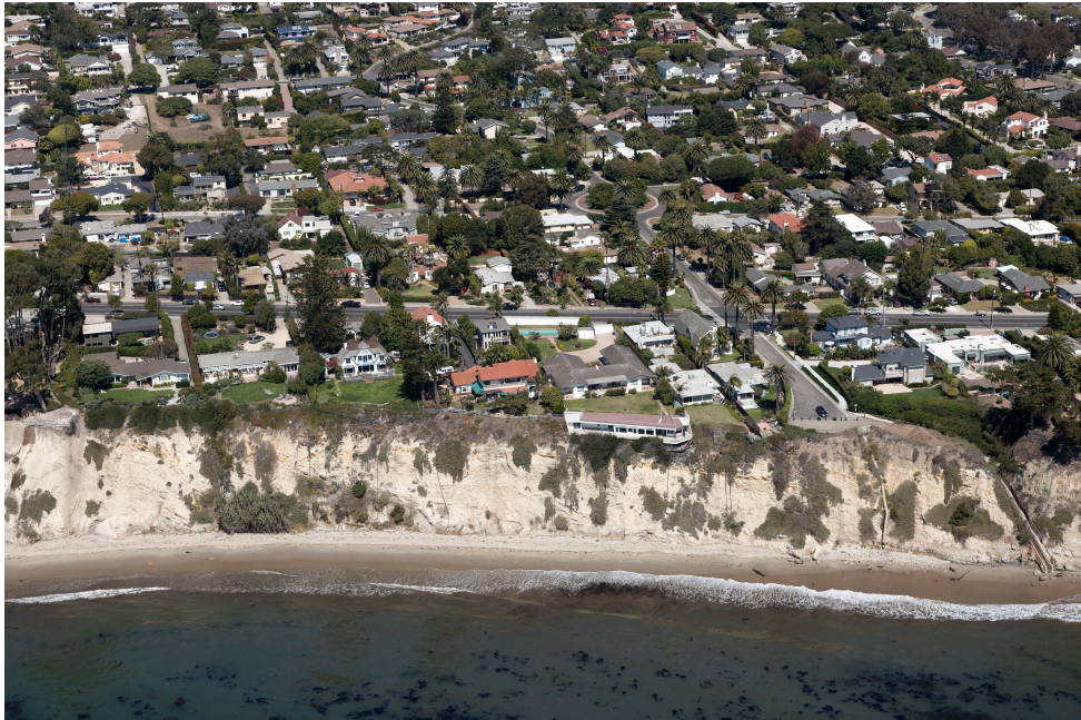
Figure 2.15 Some structures along the Mesa are virtually at the cliff's edge (photo: Kenneth and Gabrielle Adelman, California Coastal Records Project).
