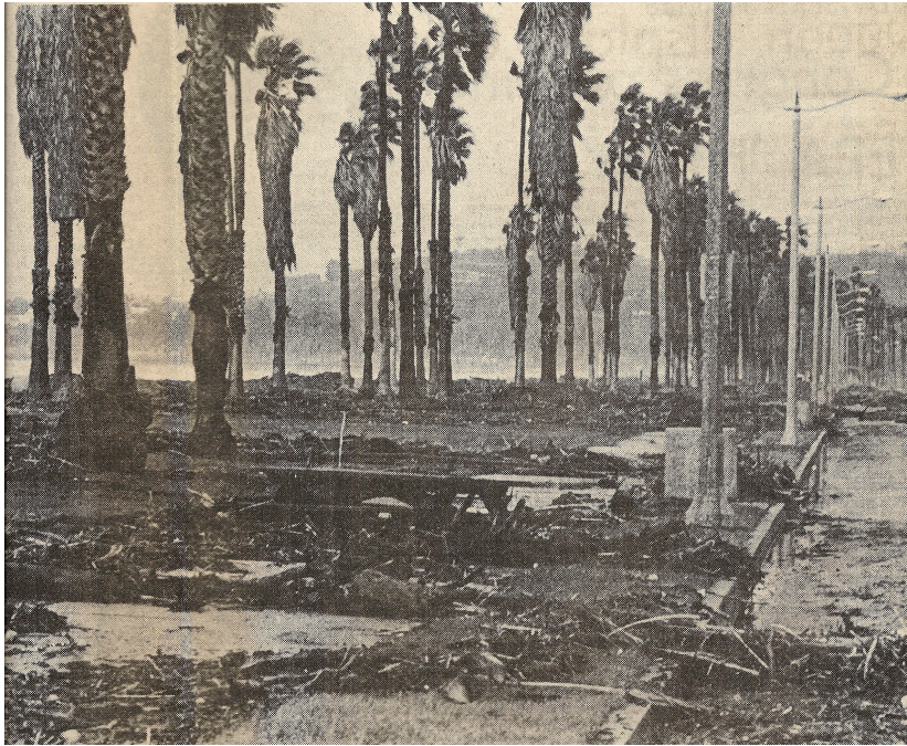
Figure 2.10 Palm Park, on Cabrillo Boulevard, was strewn with debris, including a picnic table that was carried in by waves that had overtopped East Beach in March 1983 (source: Santa Barbara News-Press).
