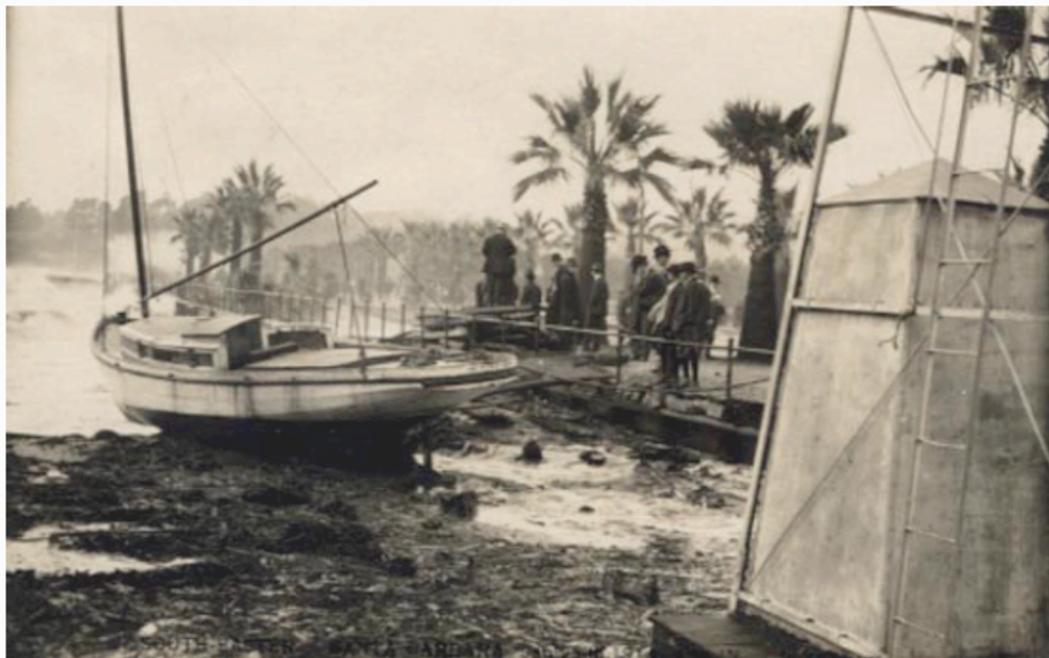
Figure 2.18 A boat was beached against a seawall just west of Stearns Wharf during the storms of 1914.
