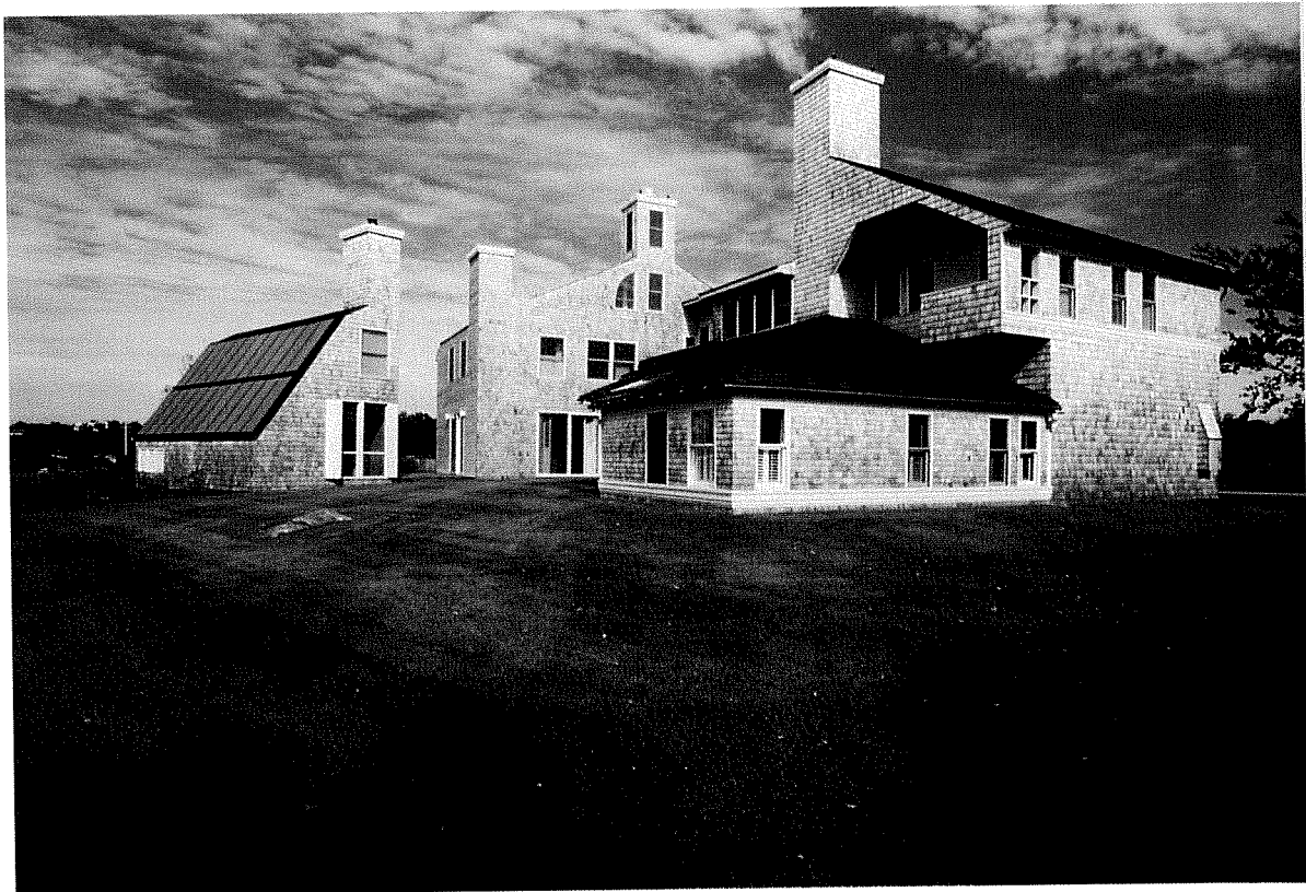
The image of a building can also derive from its climate. For example, the Shattuck House, on the Connecticut shore, responds to its New England climate with an active solar heat system housed on the roof of a small summer cottage. The cottage is separated from the main house at such an angle as to funnel the predominantly southwesterly breezes into the courtyard and house during the steamy hot summers. Above: Village in Switzerland. (Jeff Riley) Right: Shattuck House. (Norman McGrath)
