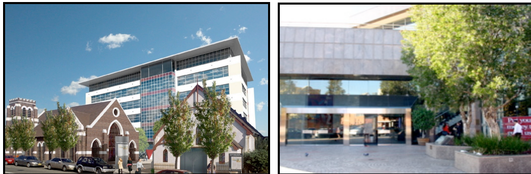
Figure 9. Kogarah Town Square: Sydney, Australia. Traditional architecture, central rail stations, and open civic squares.
