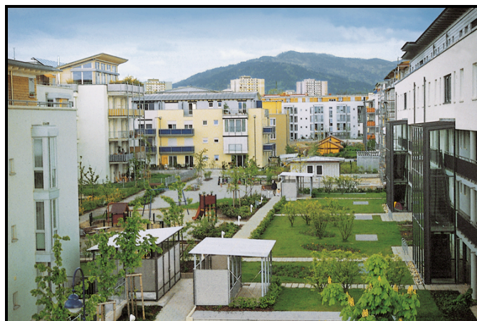
Figure 1. Green TOD in Rieselfeld, Germany: Gardens and play areas replace surface parking.
