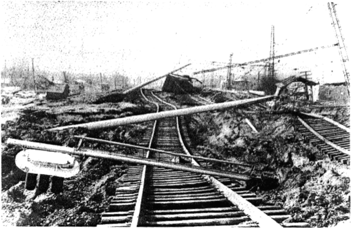
FIG. 13. Photograph of Failed Embankment at Railway Station in Nalband (Site 3) (Photo Courtesy of A. Karakhanian, 1989)
