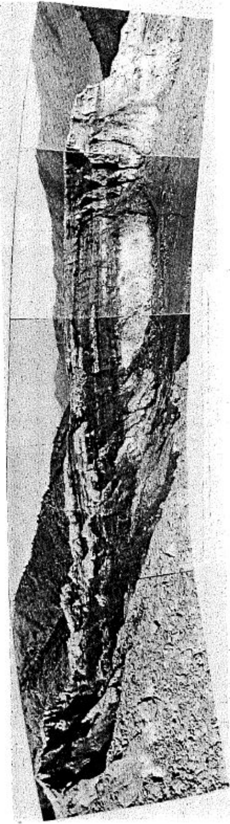
Figure B.6.3(a): Photograph showing post-failure conditions at the Old Dam; photo taken looking upstream towards the back edge and the "horseshoe shaped" scarp (Dobry and Alvarez, 1967).
