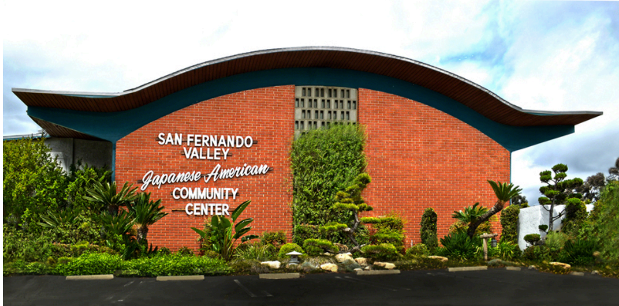
Figure 3.3 The San Fernando Valley Japanese American Community Center, 2013. The original gymnasium pictured here was built in 1959 and exists today. Courtesy of the SFVJACC.
