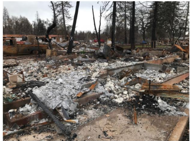
(b) Structures burnt by fire
