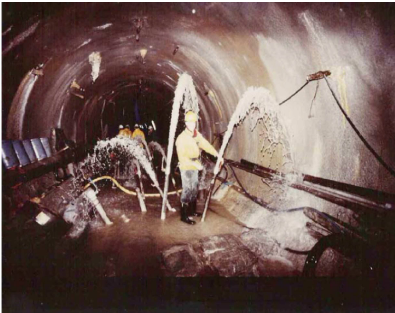
Fig. 4.10. Water inflows during LEP tunnel construction.
