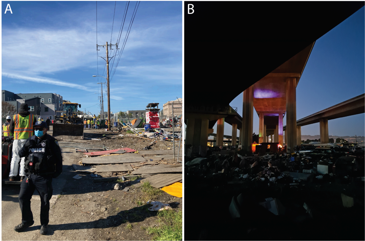
Figure 7. (A) The final stages of destruction of the Wood Street encampment on April 20, 2023. The lead author was onsite bringing food and water to partners and collaborators working in the encampment when hundreds of riot police and demolition crews swept into the camp. At one point, an estimated 250 people lived at the site. (B) A photo from under the freeway overpass where the “Cob On Wood” community project was constructed, taken during a community celebration. The lights from the party warmly frame the cob kitchen, free store, and health clinic. The overpass acts as a kind of great hall, echoing and uplifting the sounds of music alongside the clatter of food, laughter, and conversation.
