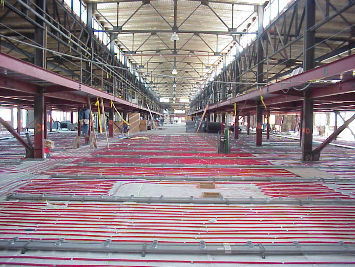
Figure 7.4 Radiant system (WSP Flack and Kurtz 2007).
