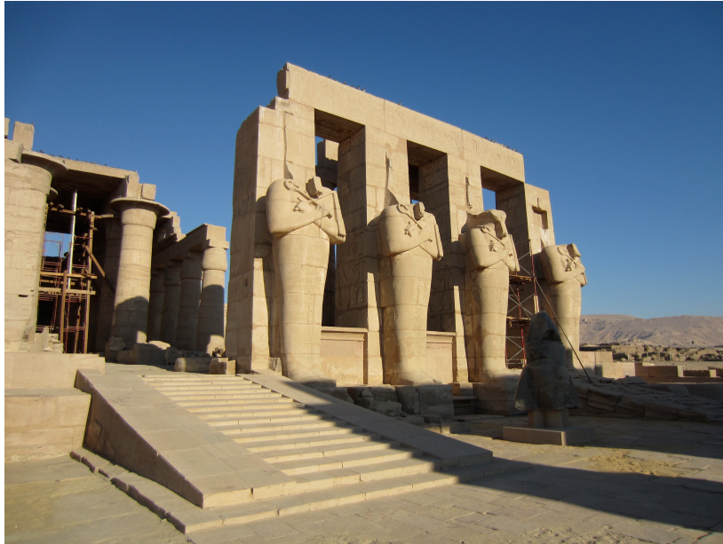
Figure 38. Central Ramp Leading from the Second Courtyard into the Hypostyle Hall of the Ramesseum. Photo by Author.
