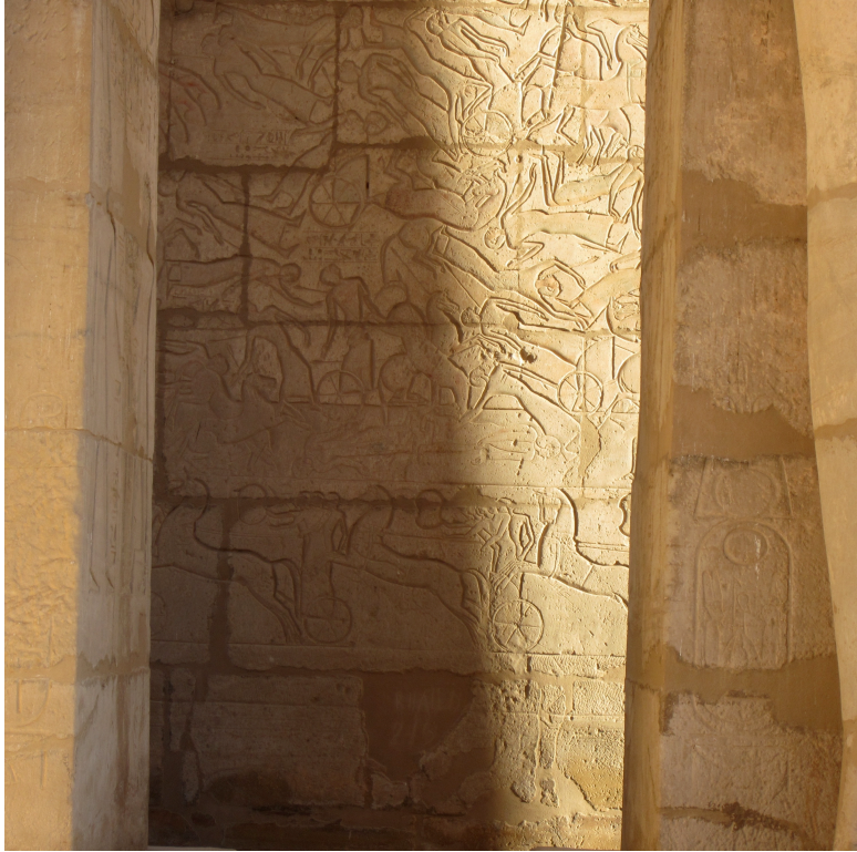
Figure 30. Central Opening in between Osiride Pillars onto the Northern Wing of the Second Pylon of the Ramesseum. Photo by Author.
