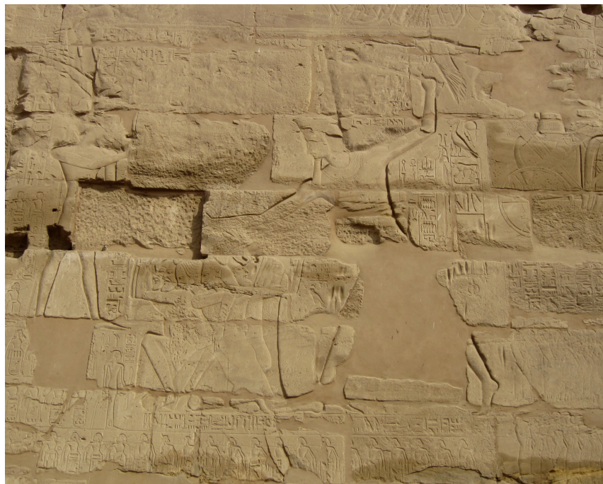
Figure 53. Triumphal Relief of Ramses II on the Eastern Side of the Southern Exterior Wall of the Hypostyle Hall of the Temple of Amun at Karnak. Photo by Author.
