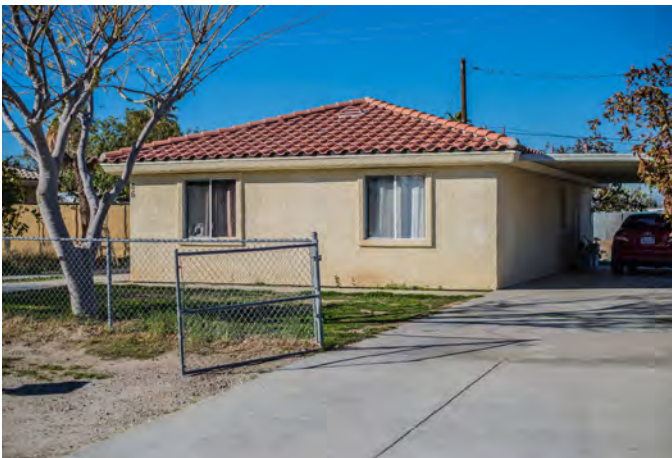
Figure 16. Stick Built Home in Thermal
