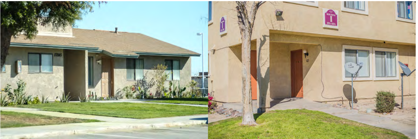
Single story apartment complex in Thermal
