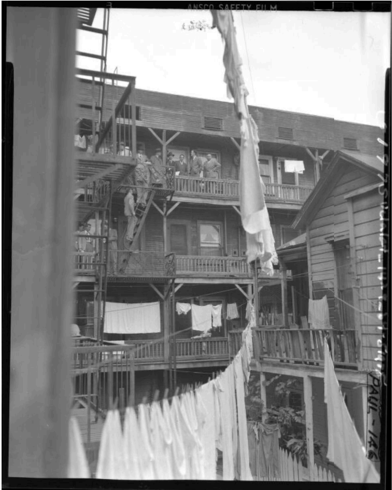
Figure 8: “Housing Director Holtzendorff and men going up rickety fire escape of tenement during tour of slum areas in Los Angeles, Calif., 1948.”
