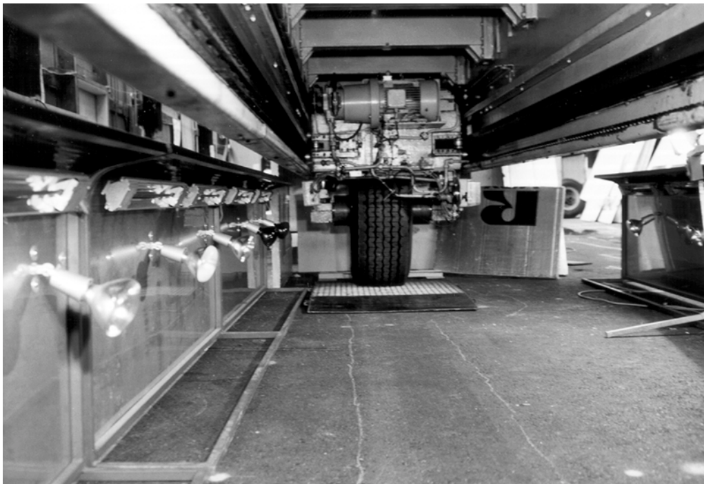
Figures 9a and 9b. Aluminum reflector with resistance-heating element and infrared lamps.
