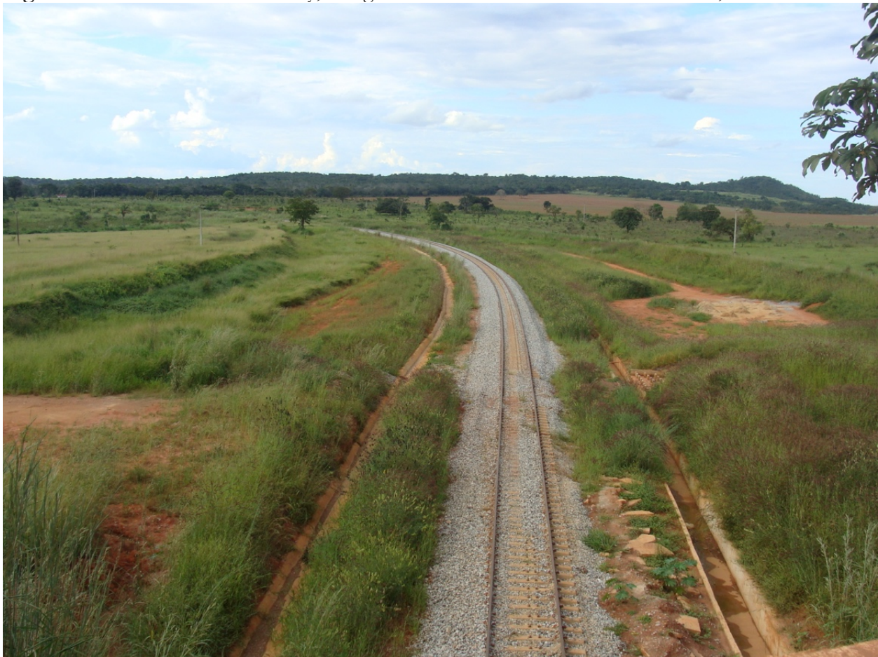
Figure 1. The North-South Railway, inaugurated but almost unused in Goiás state, 2014
