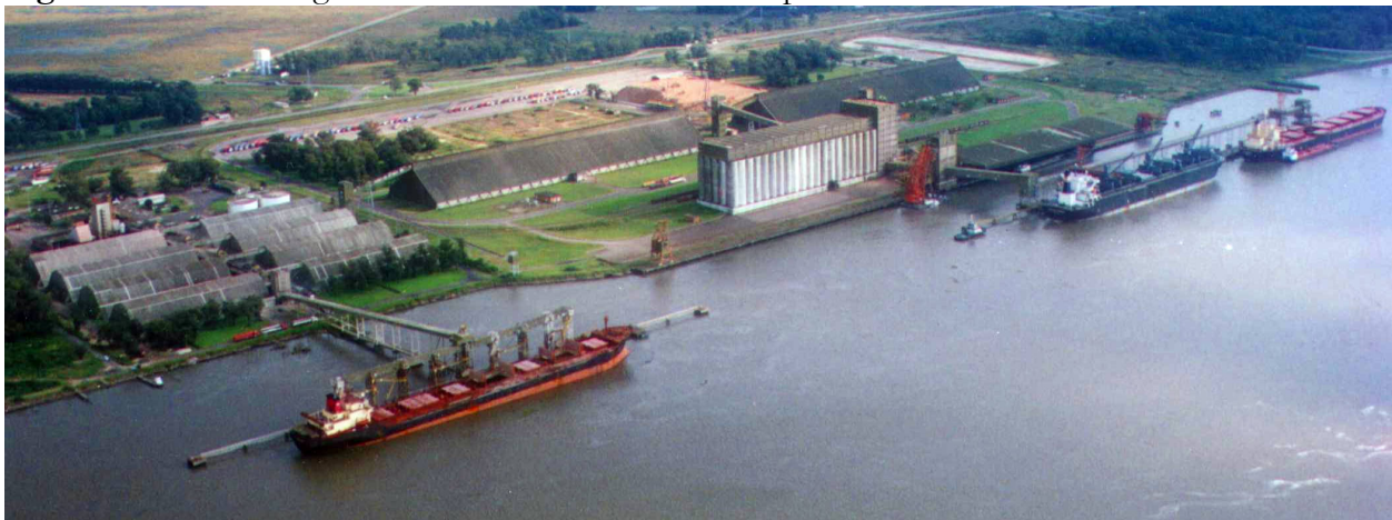
Figure 6. The CCGL grain terminals at the Rio Grande port
