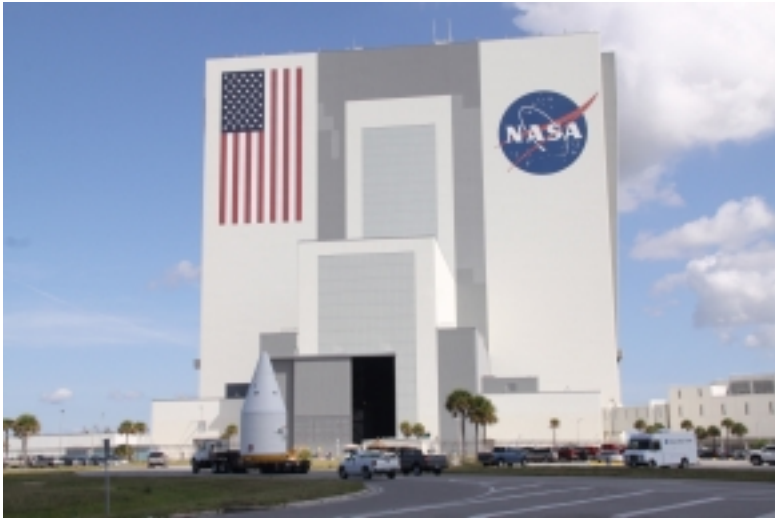
Fig. 13: U.S. FLAG AND THE NASA INSIGNIA AFTER THE VEHICLE ASSEMBLY BUILDING WAS REPAINTED
