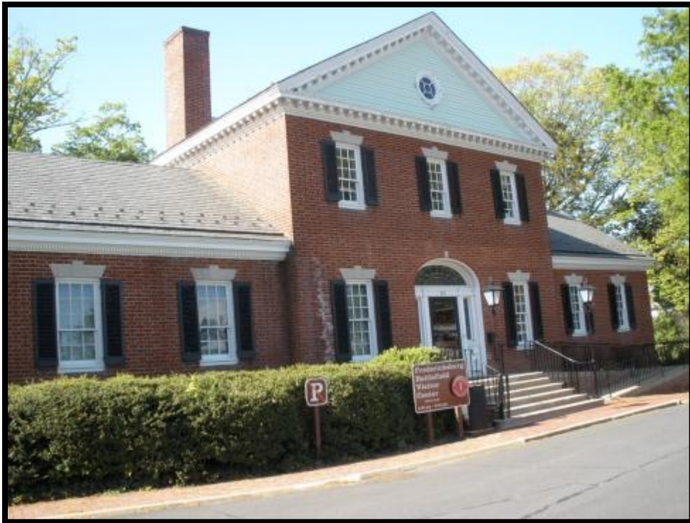
(Figure 4.19) The Fredericksburg Visitor Center. Photo by Susan C. Hall, 2010.
