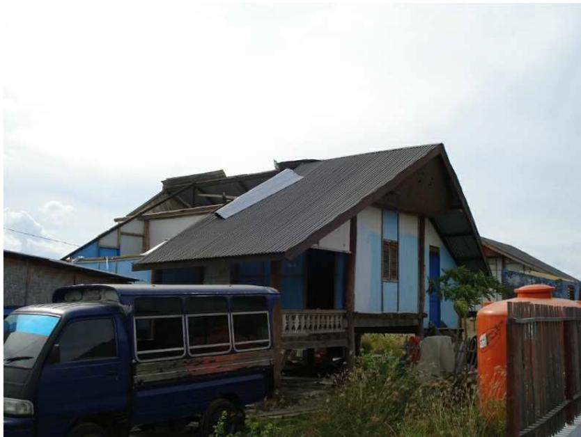
**Figure 5.9: A house in Gampong Jawa with a missing roof due to strong winds less than two years after its construction had been completed**
