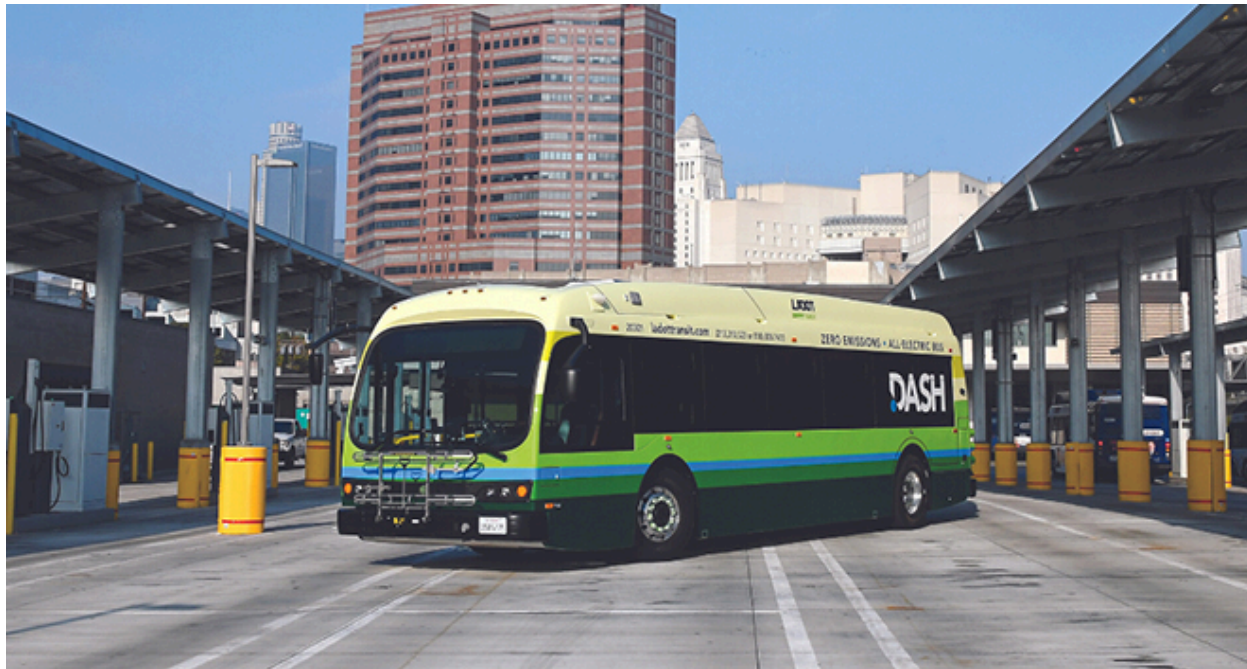
LADOT solar-powered bus depot.
