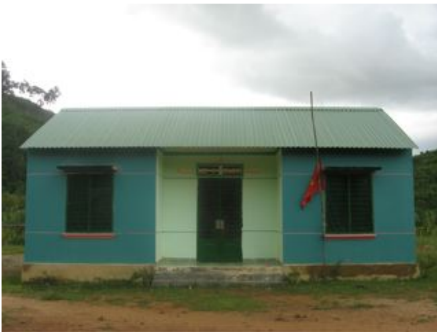
Photo 16: Standard house built for resettled families
