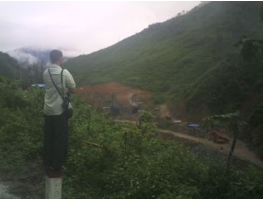
Photo 2: Building new roads to construction sites for A Vuong Dam
