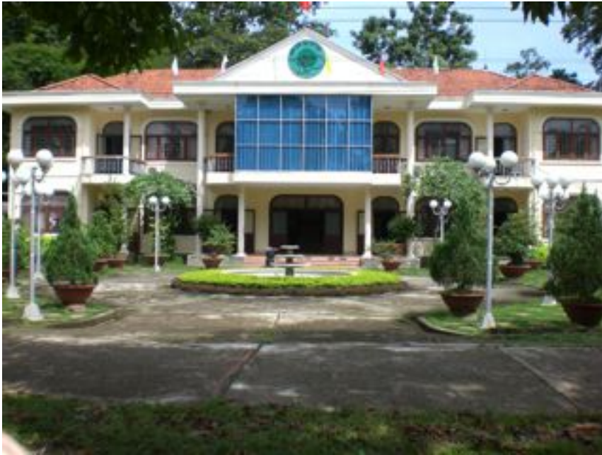
Photo 13: Cat Tien National Park Head Office
