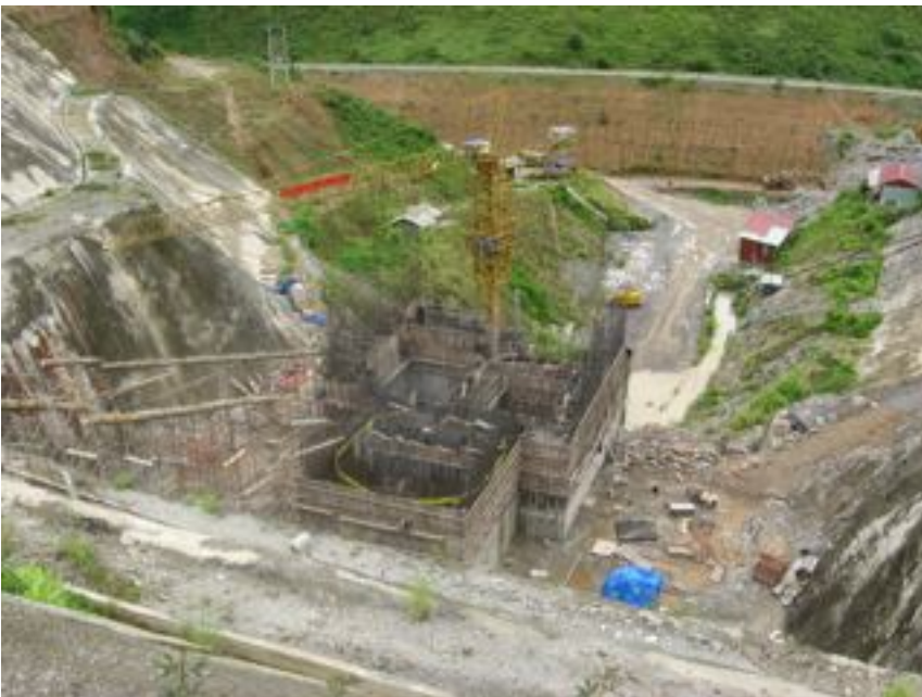
Photo 4: The dam wall and entrance to the tunnel that diverts the river water through electricity-generating turbines and then back into the river bed several km downstream
