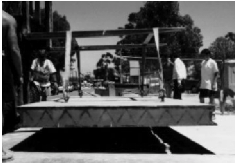
Figure 3.7: Field installation of a FRP Composite Deck Panel [Zhao, 1999].
