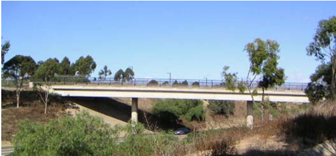
Figure 9.1a: Elevation View of Voigt Drive / I-5 Overcrossing Taken from South-West side of the Bridge
