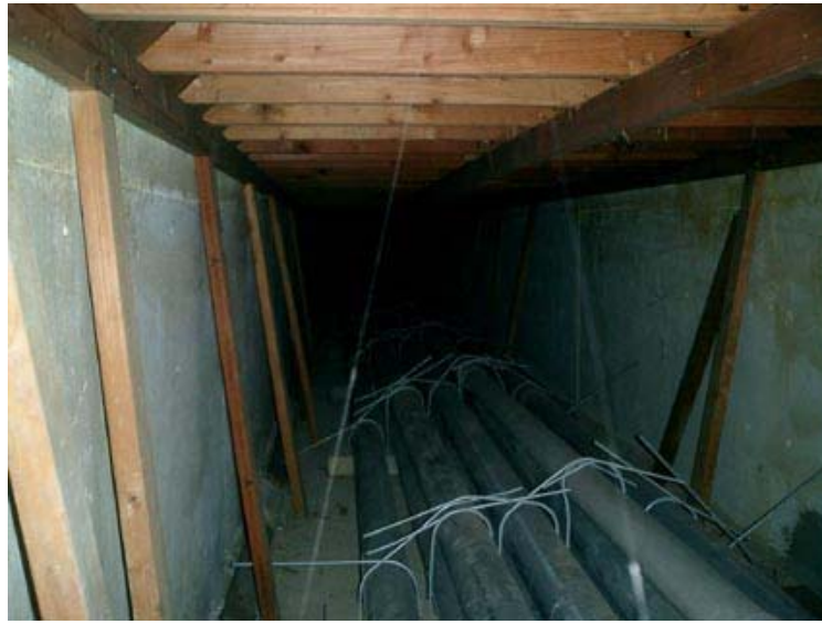
Figure 9.5: Interior of Northern-Most Cell of Voigt Bridge
