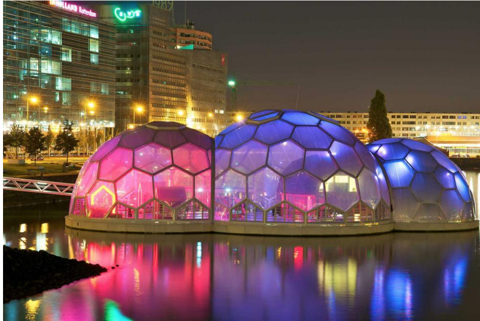
Fig. 5. The Floating Pavilion (2005-2010). Three interlinked spheres, the largest of which with a radius of 12 meters. The total floor space of pavilion island is 46 x 24 meters. An innovative and sustainable building, which is climate change resilient and reflects Rotterdam's adaptation strategy in response to climate change. Now that all commercial and industrial activity has been moved to massive transfer sites at the coast, the question remains of how to re-appropriate vacant former city harbors? Rotterdam's residents were previously so strongly connected to the harbor activities. How will they be involved with the waterfront in the future?
