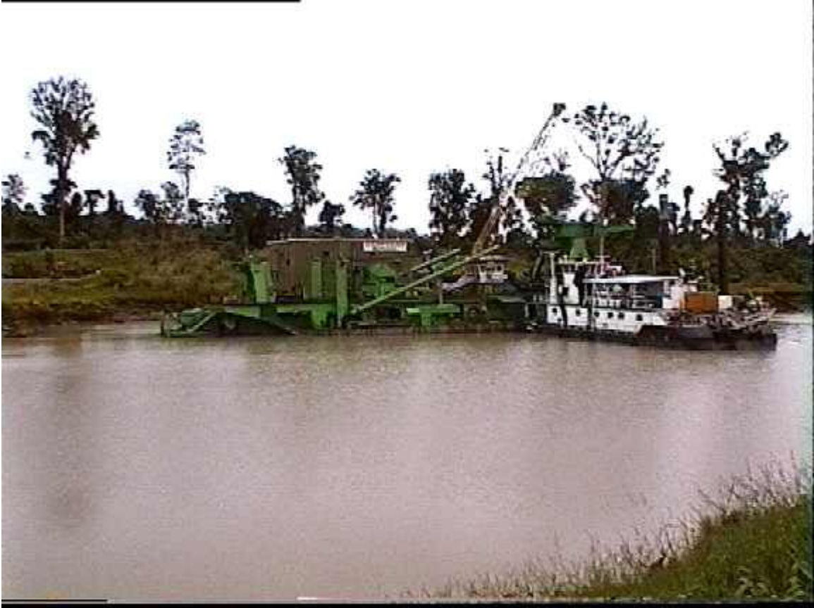
Figure 6. Slot dredger on the Ok Tedi River (Kehdingen, 2001).
