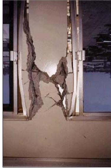
(b) Interior up-close view of the column damage caused by the earthquake
