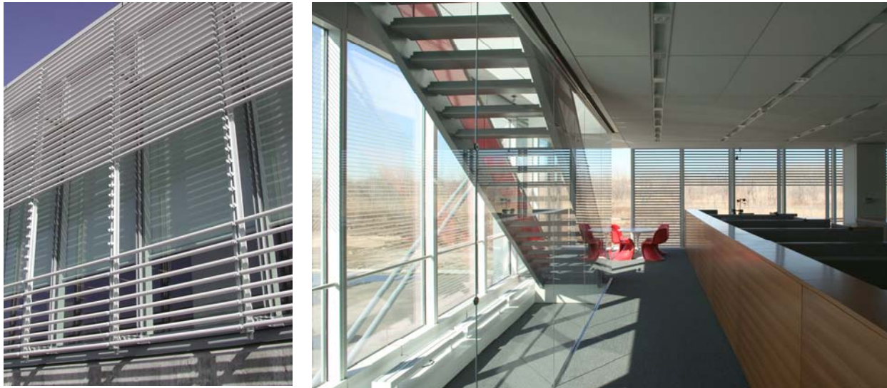
Fig. 1. Exterior view of the west façade of The New York Times daylighting mockup (left) and interior view of Area B (right) on February 23, 2004 with south-facing windows on the left-hand side of the photograph.
