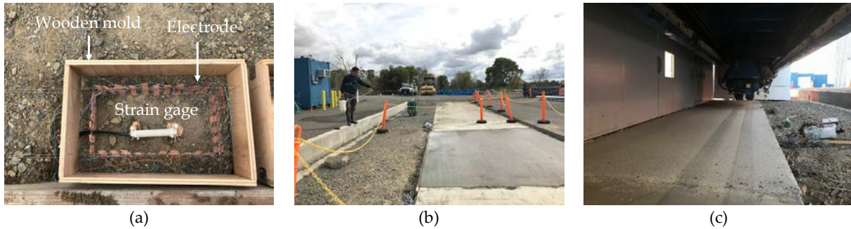
Figure 4. (a) The wooden mold for casting the self-sensing concrete regions, along with the electrodes mounted on fishing wires and strain gages, are shown. The picture of concrete slab (b) immediately after casting and (c) after 28 days of curing are shown.
