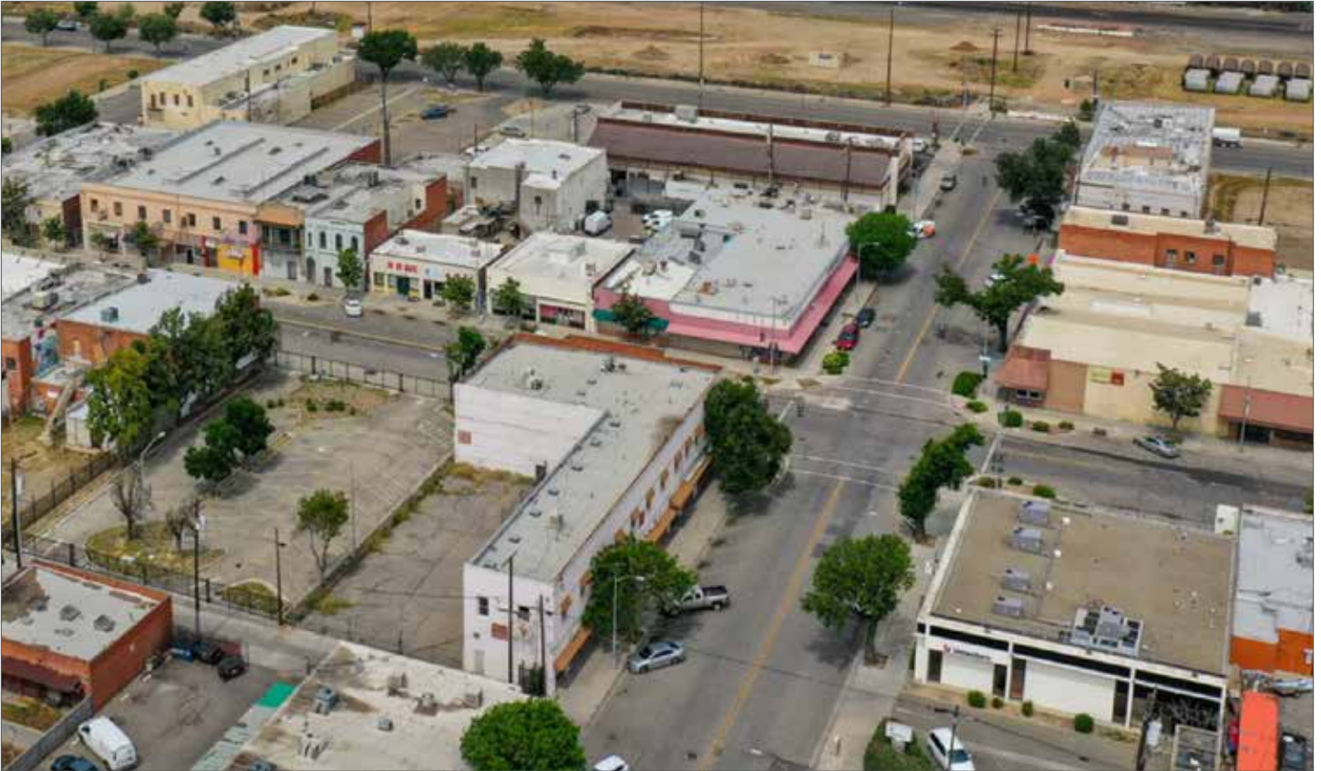
Historic Chinatown at Kern Street and F Street, where several TCC and leveraged projects will come to fruition.
