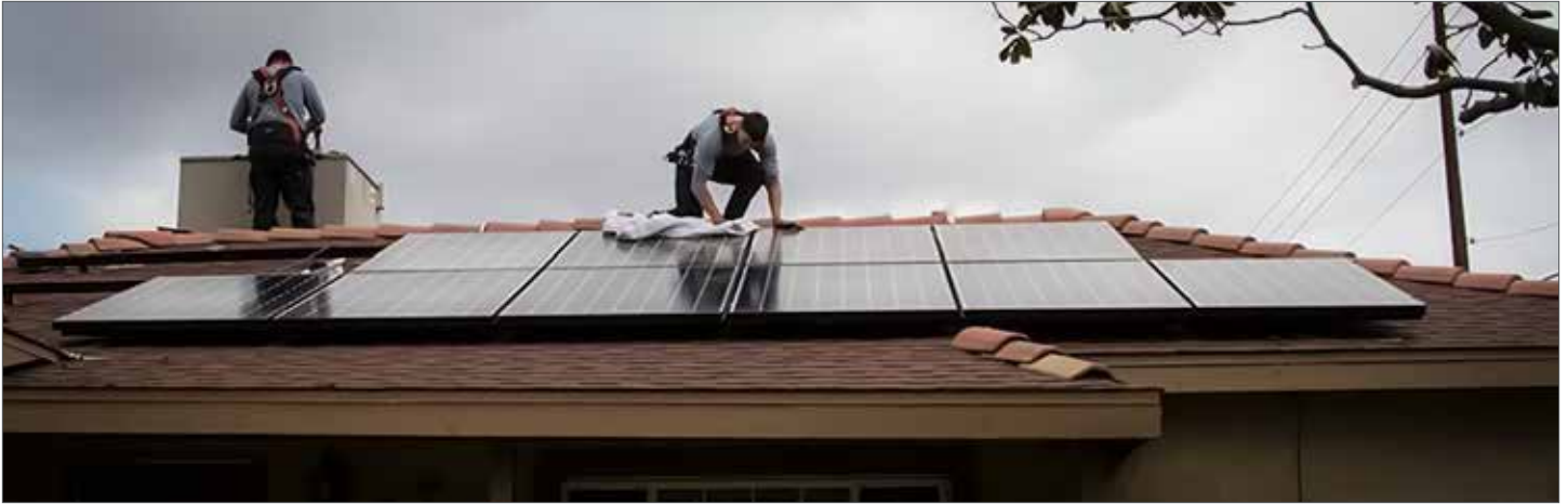
A Fresno EOC crew installs solar panels on a single-family home. Photo credit: Fresno EOC
