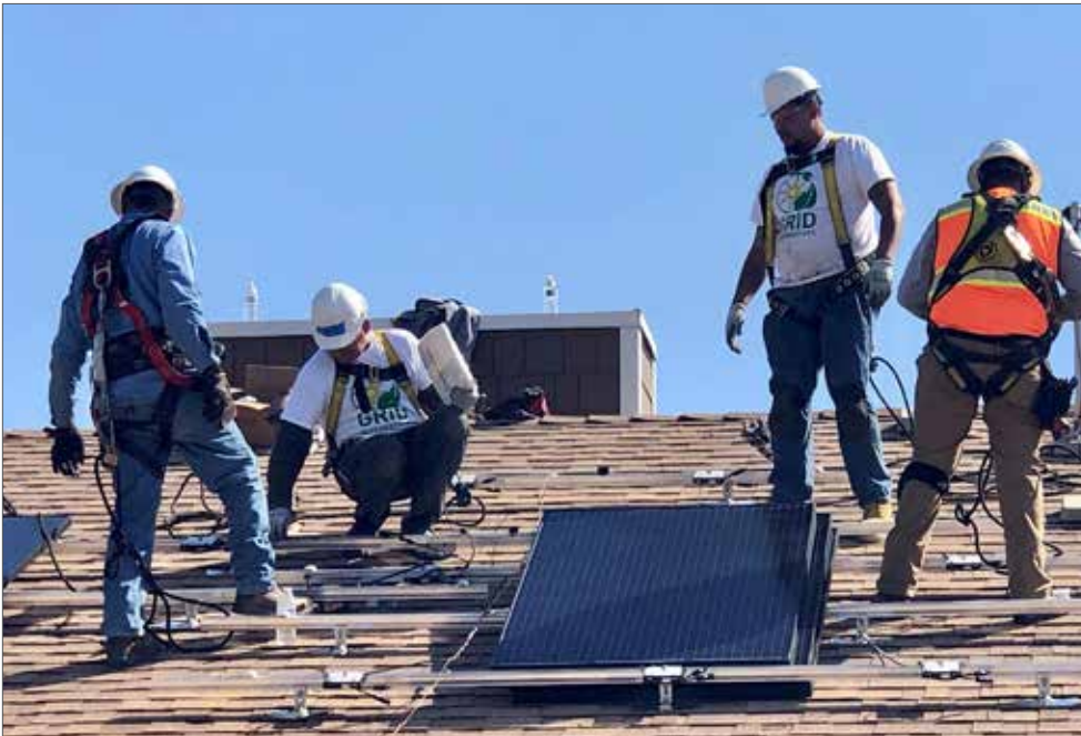
A GRID Alternatives crew installing solar panels on the Bridges at Florence affordable senior living apartments in the Transform Fresno project area. Photo credit: Fresno Housing Authority
