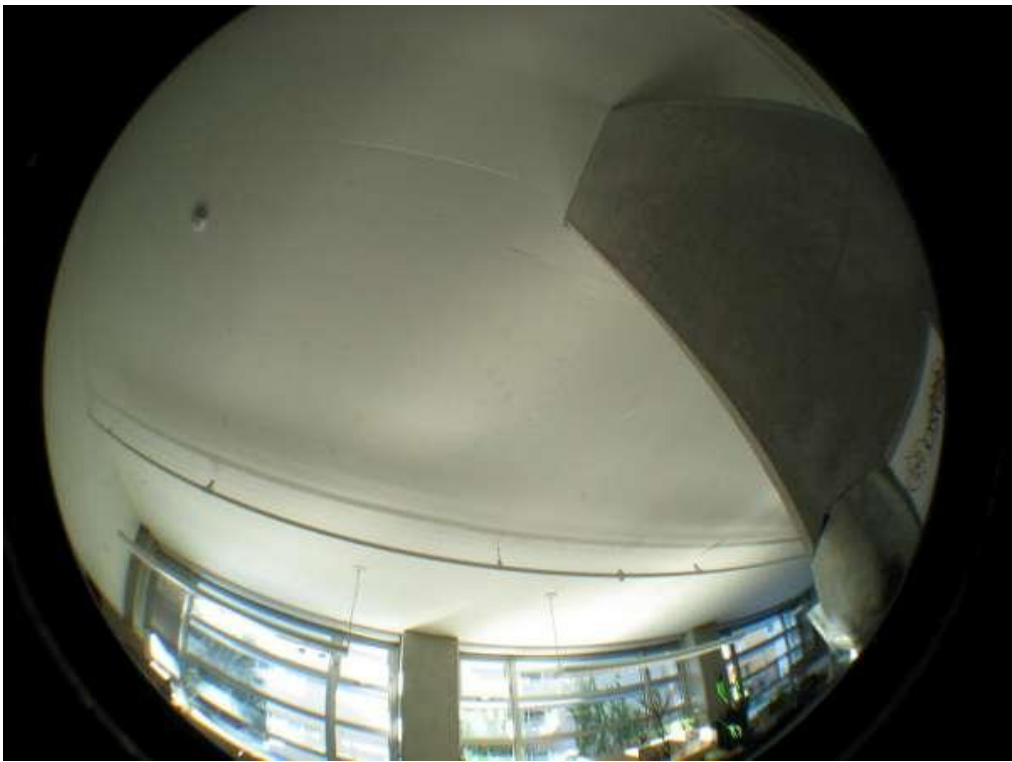
Figure 38 Fisheye lens photo of upper portion of facade and ceiling
