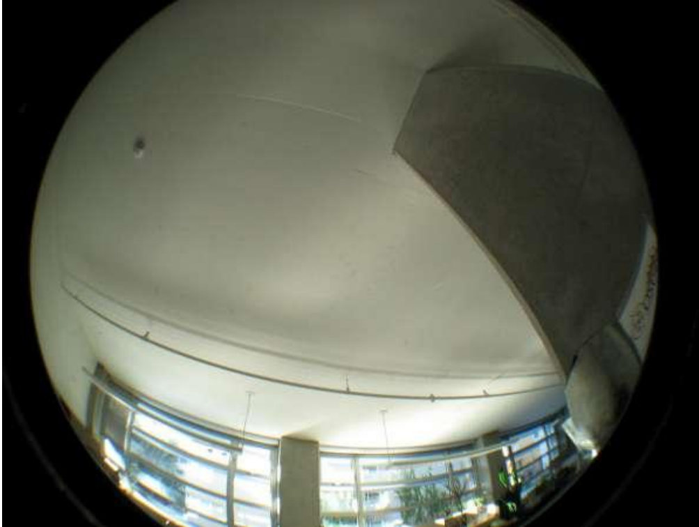
Figure 59 Fisheye lens photo of upper portion of facade and ceiling
