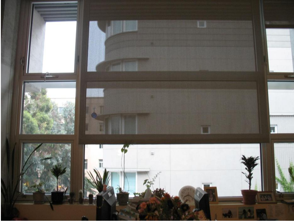
Figure 24 Interior roller shades in a south-facing 3 rd floor suite
