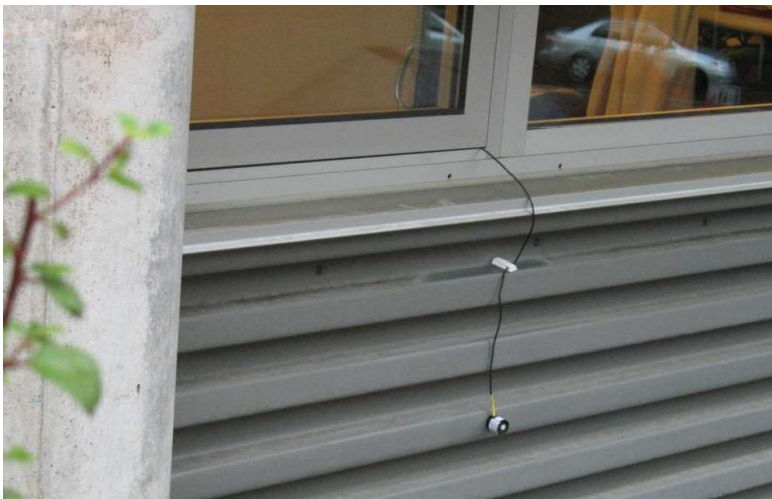
Figure 45 Sensor used to measure vertical illuminance on the facade
