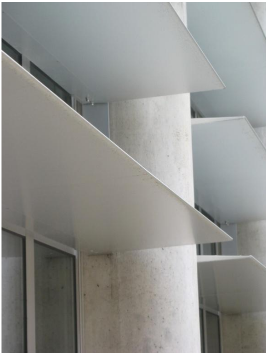
Figure 9 Detail of aluminum louvers
