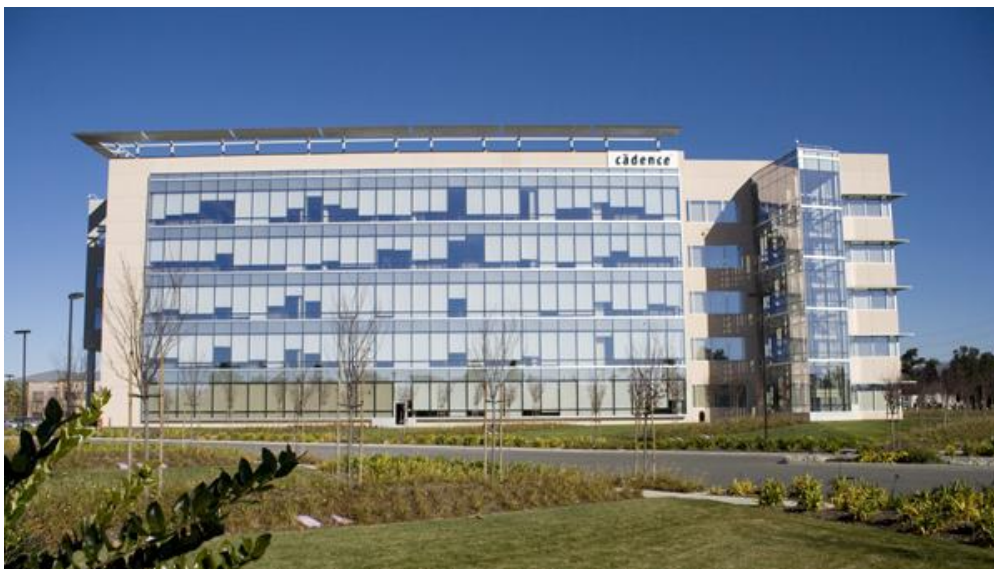
Figure 1 Highly-glazed office building in San Jose. View of west elevation, December 2009.
