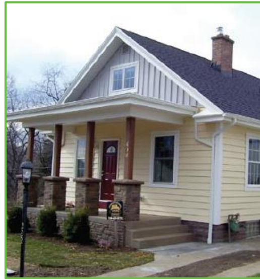
Asdal Builders achieved a HERS* score of 65 and cut energy use by 80% with a gut-rehab of this 1930s-era Pittsburgh home.
