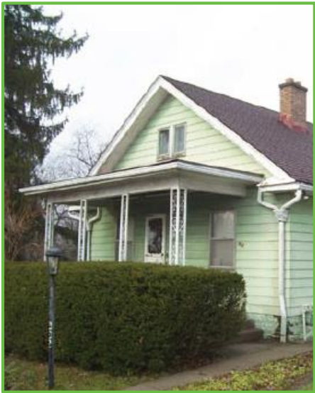
Pittsburgh home pre-retrofit
