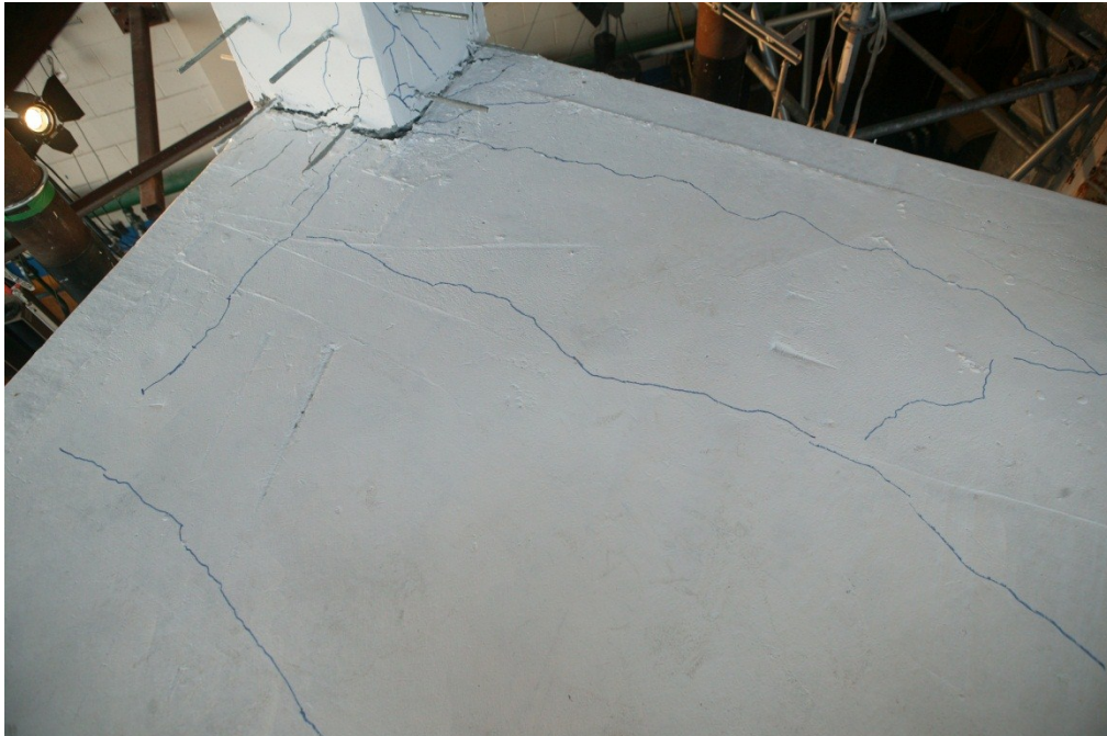
Figure 7.149 Crack pattern of slab in specimen U-J-2
