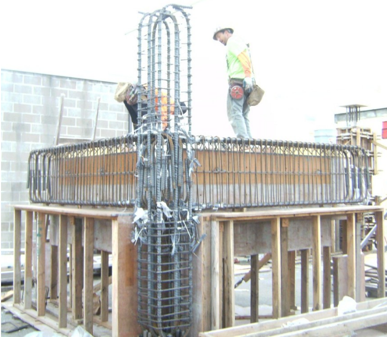
Figure 6.8 Reinforcement cage of specimen U-J-2
