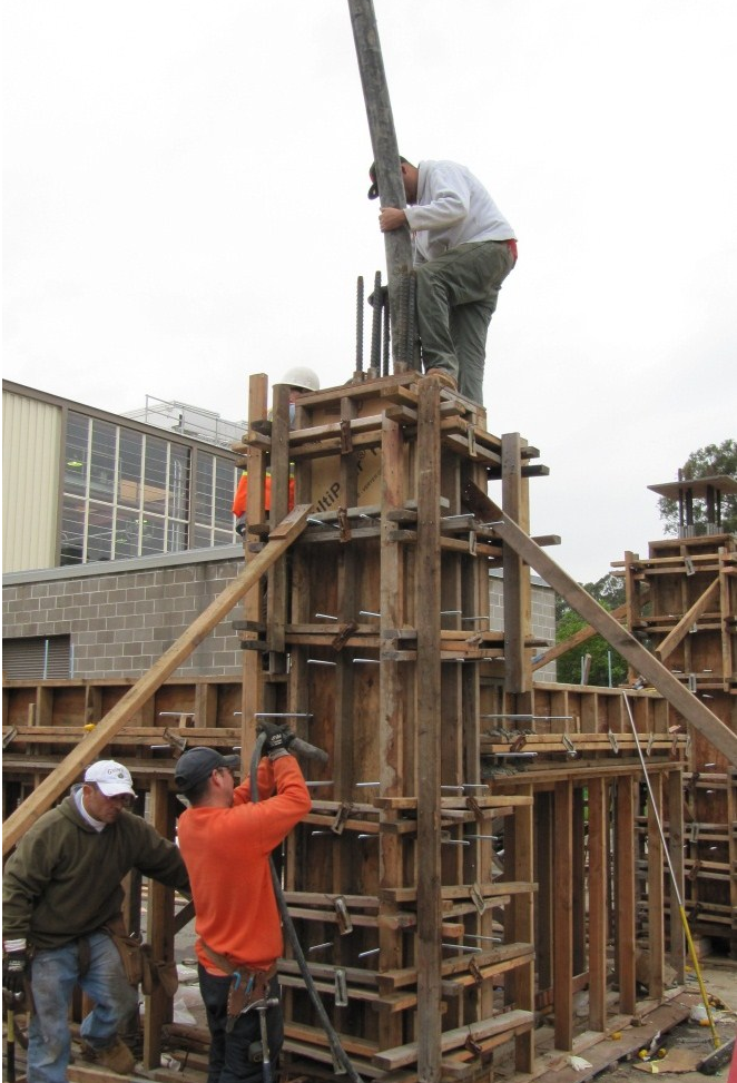
Figure 6.10 Concrete casting and compaction of test specimens
