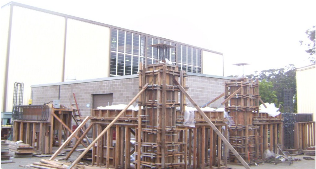
Figure 6.12 Cast specimens curing and finalized formwork and scaffolding
