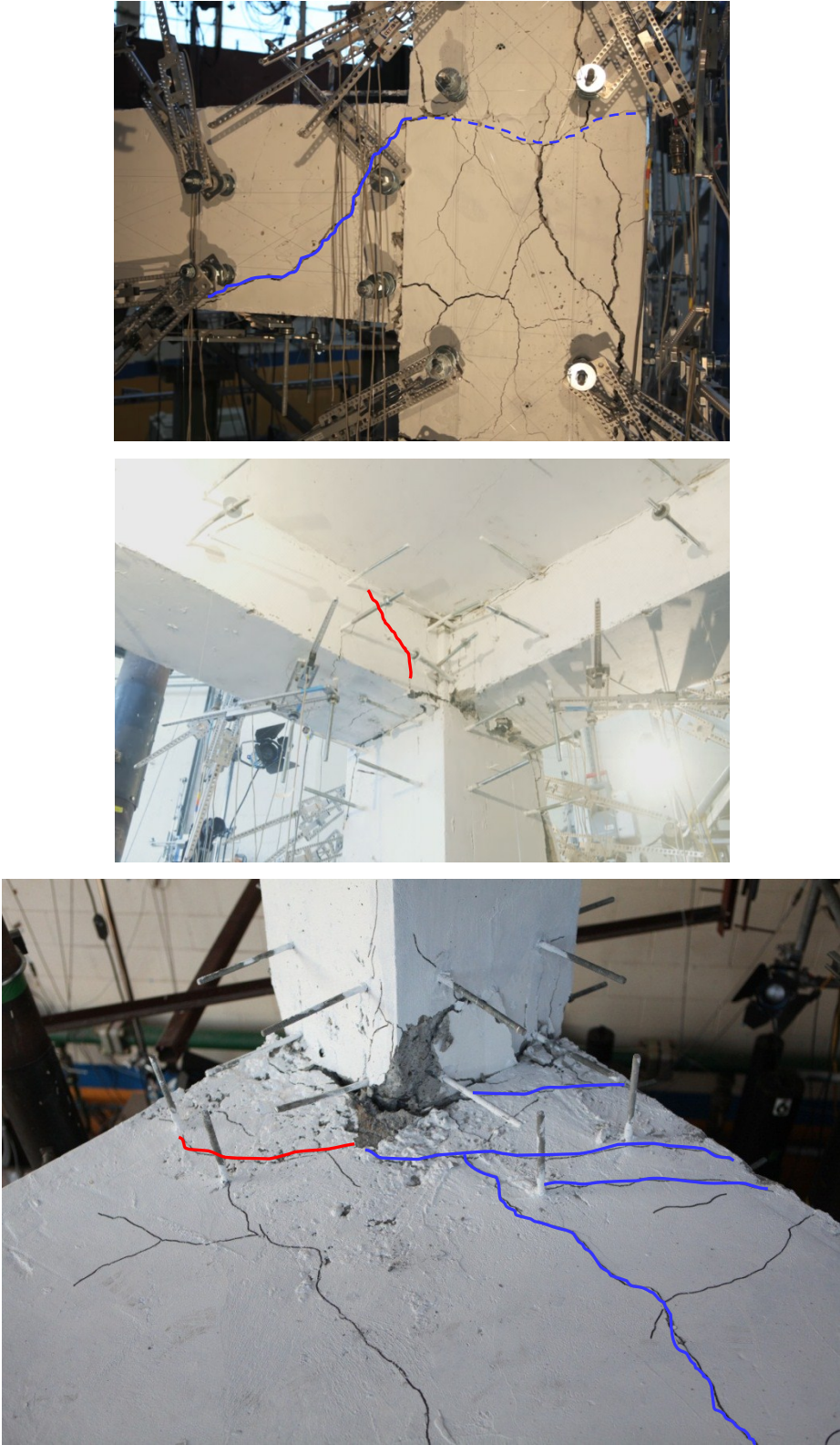
Figure 7.140 Torsional cracking in specimen U-BJ-1
