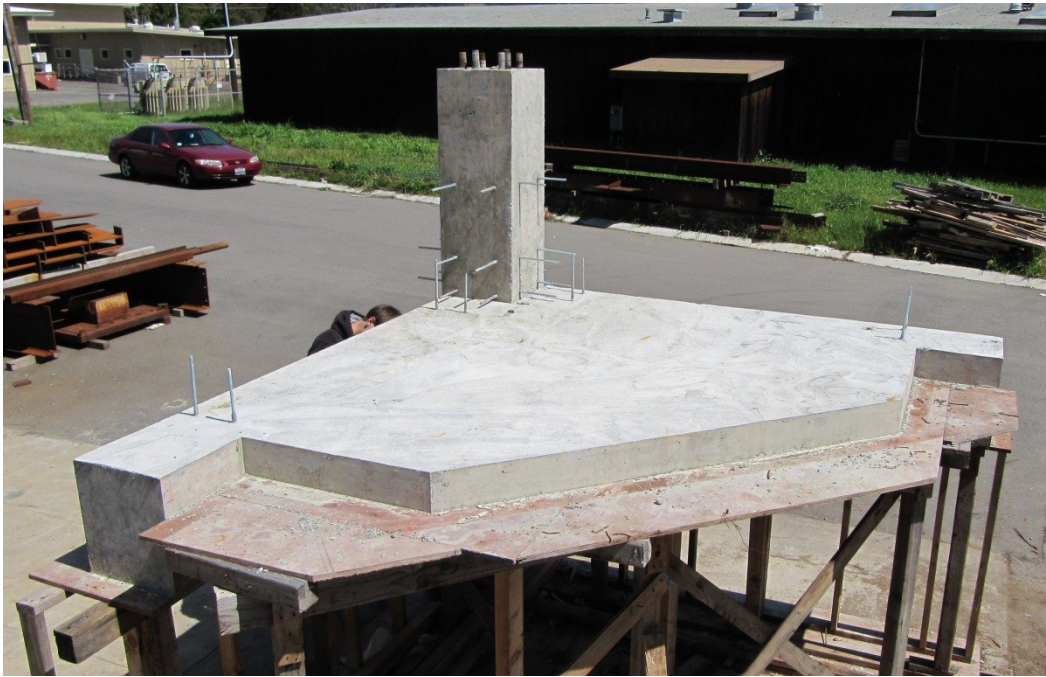
Figure 6.13 Finished test specimens after removing wood forms
