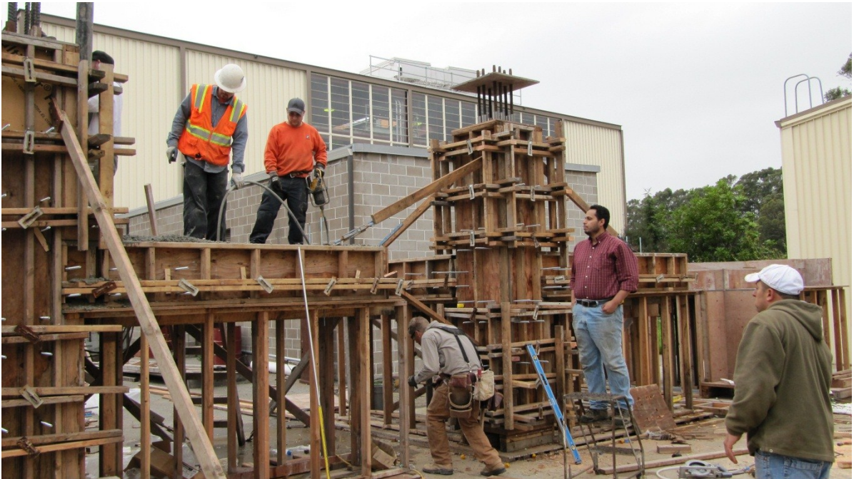
Figure 6.11 Supervision of concrete casting and compaction
