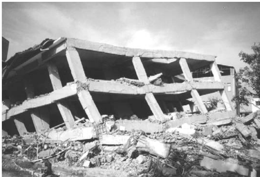
Figure 2.4 Collapsed building following Izmit, Turkey earthquake of Aug. 17, 1999, Said and Nehdi [130]
