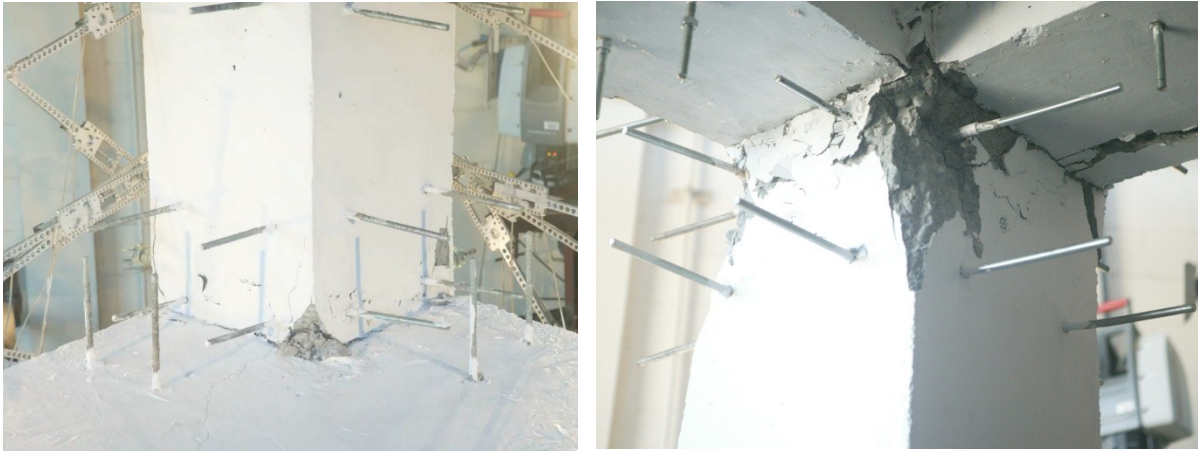
Figure 7.49 Evidence of 3D shear diagonal strut through the joint of specimen B-J-1
