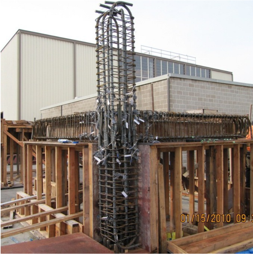
Figure 6.6 Steel cage construction of specimen U-J-1
