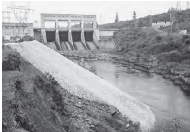
Figure 16. Gravel augmentation via high-flow stockpile on the Sacramento River, below Keswick dam (photo by Kondolf, 1990).
