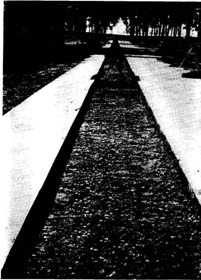
Figure 4.12 Excavated roadway trough
