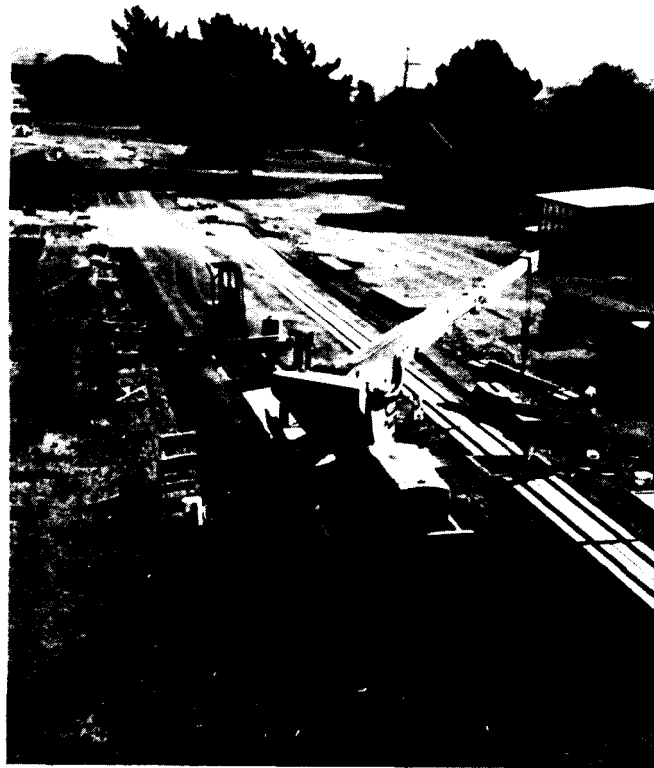
Figure 1.8 Placing roadway inductor cores
