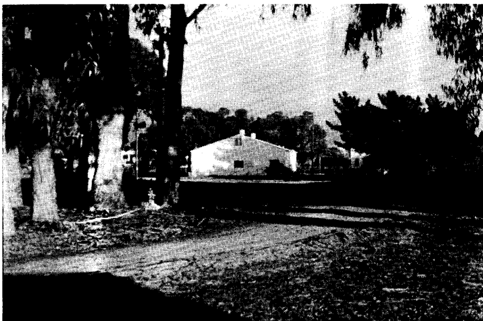
Figure 4.2 Test track site prior to construction. Photo is looking east
