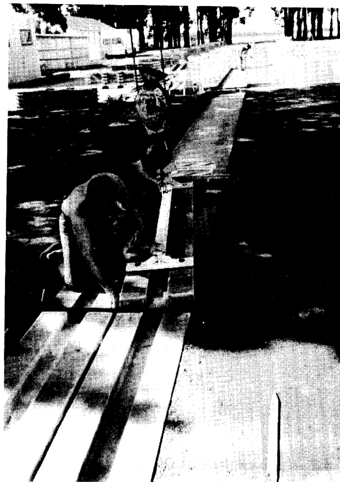
Figure 4.10 Placement of roadway modules flush with surface
