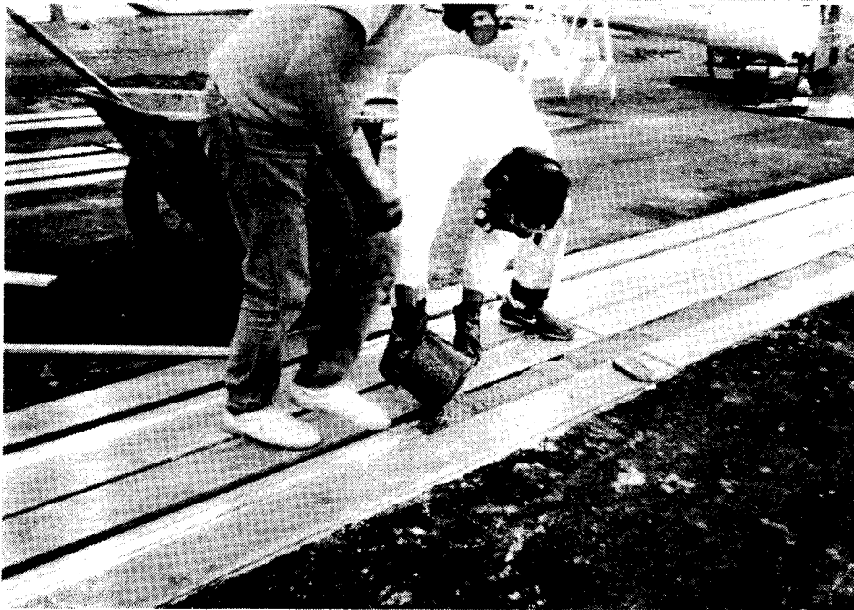
Figure 4.23 Potting busbars in place
