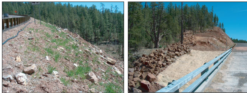
Figure 3. Alternatives to fencing to deter at-grade wildlife crossings along the Christopher Creek section of State Route 260, Arizona, USA. The steep 4:1 fill slopes below guard rails (left), boulder rip-rap (“elk-rock”) and steep cut slopes (right) were evaluated as alternative treatments to fencing.
