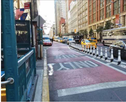
Figure 6: A bus lane separated by delineators at the intersection.
