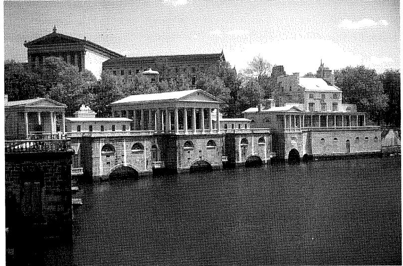
View of the Waterworks from the Schuylkill River. Courtesy Mark B. Thompson Associates.
