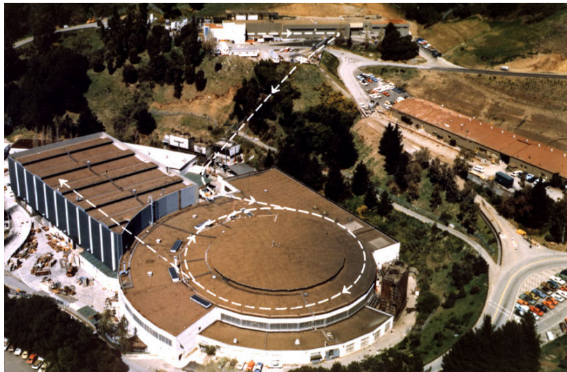
Figure 1: The Transfer Line (dotted line) brought the heavy-ion capabilities of the SuperHILAC (top) to the Bevatron, forming the Bevalac, the world's first relativistic heavy-ion accelerator.
