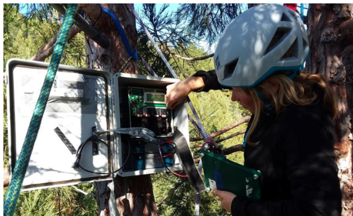
Figure 2: Monthly maintenance of equipment included retrieving acoustic data and changing batteries.
