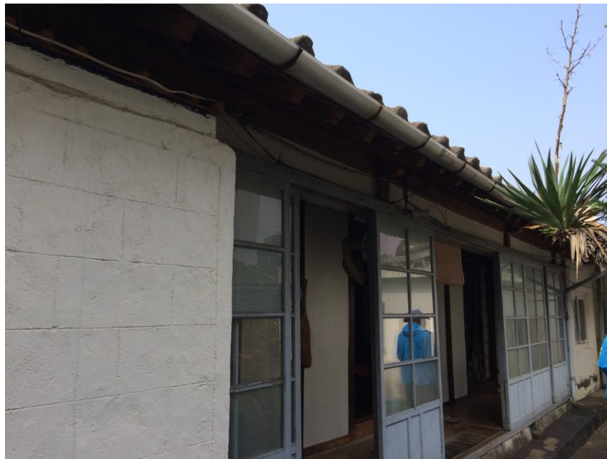
Figure 21: The Ko family house built in the 1920s. 182
