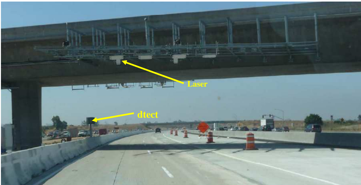
Figure 5 dtect camera position
