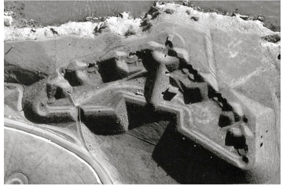
Battery Cavallo, Fort Baker, California, circa 1938. Image credit: National Archives and Records Administration, Aerial Photographs Collection, image in the public domain.
